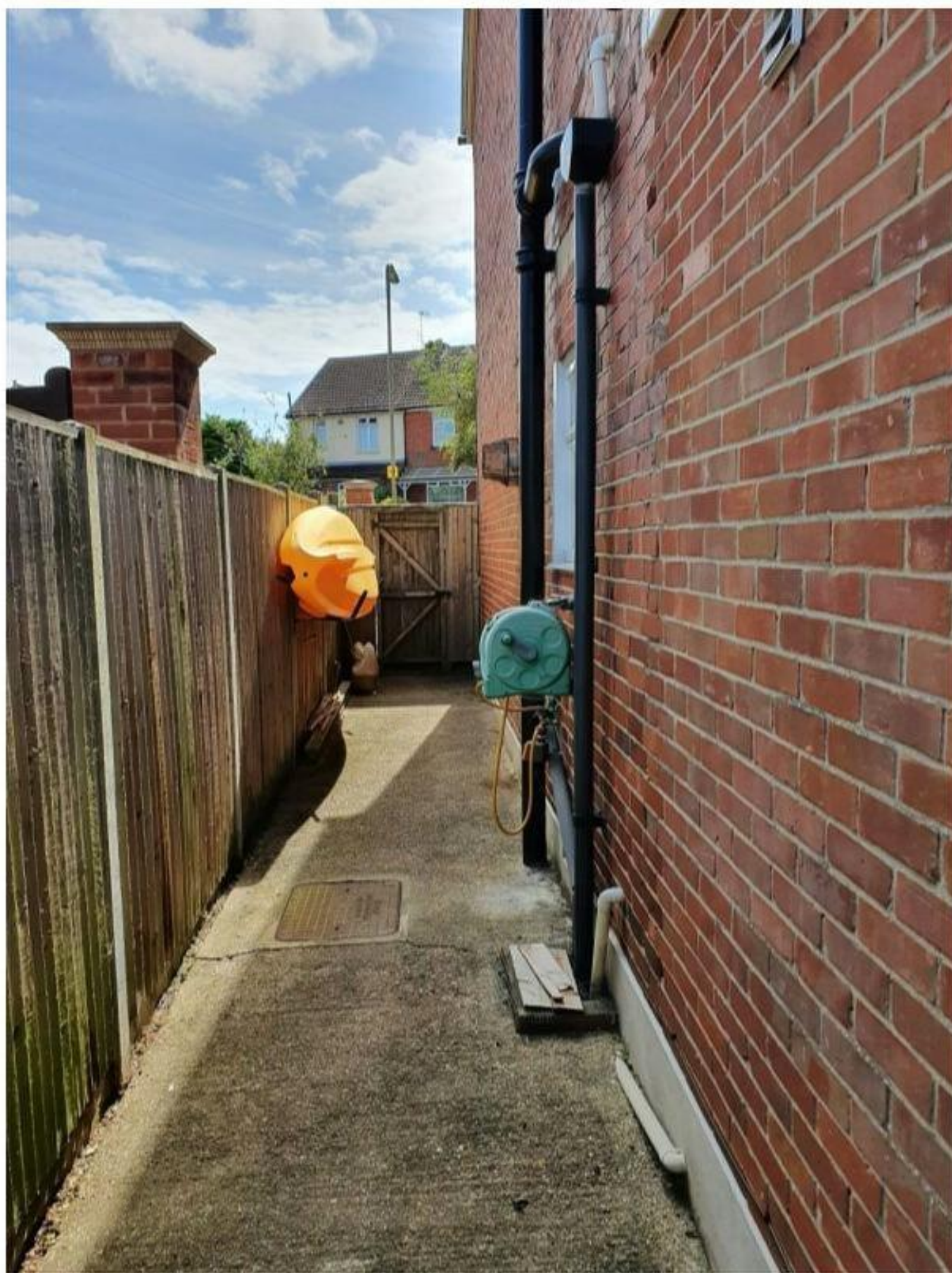
Photo 6: Side of the property looking towards the front
