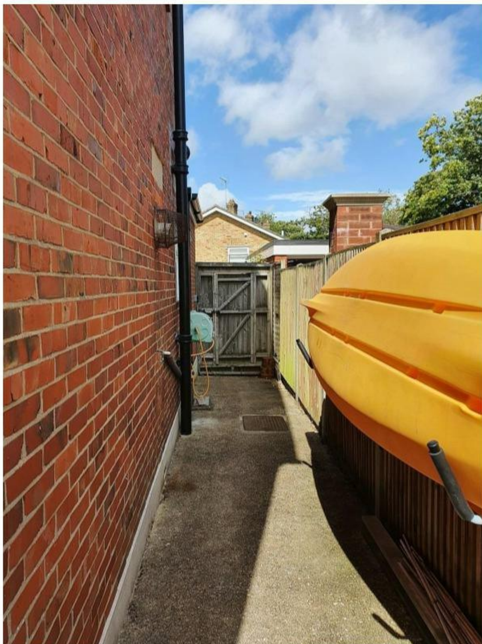
Photo 7: Side of the property looking towards the rear
