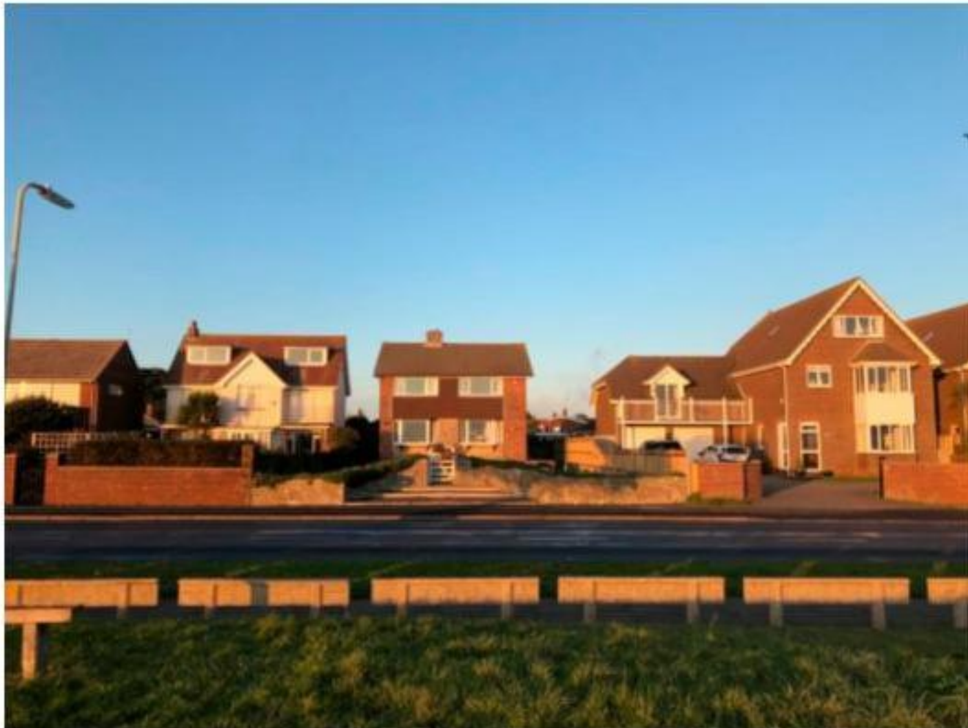
134 Sea Front southern elevation – 134a to the east and 136 to the west
