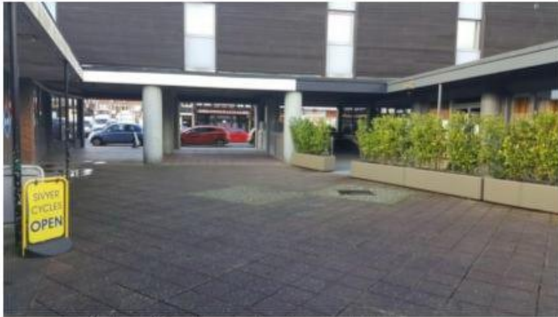
Photograph 2: Existing Undercroft Pedestrian Walkway
