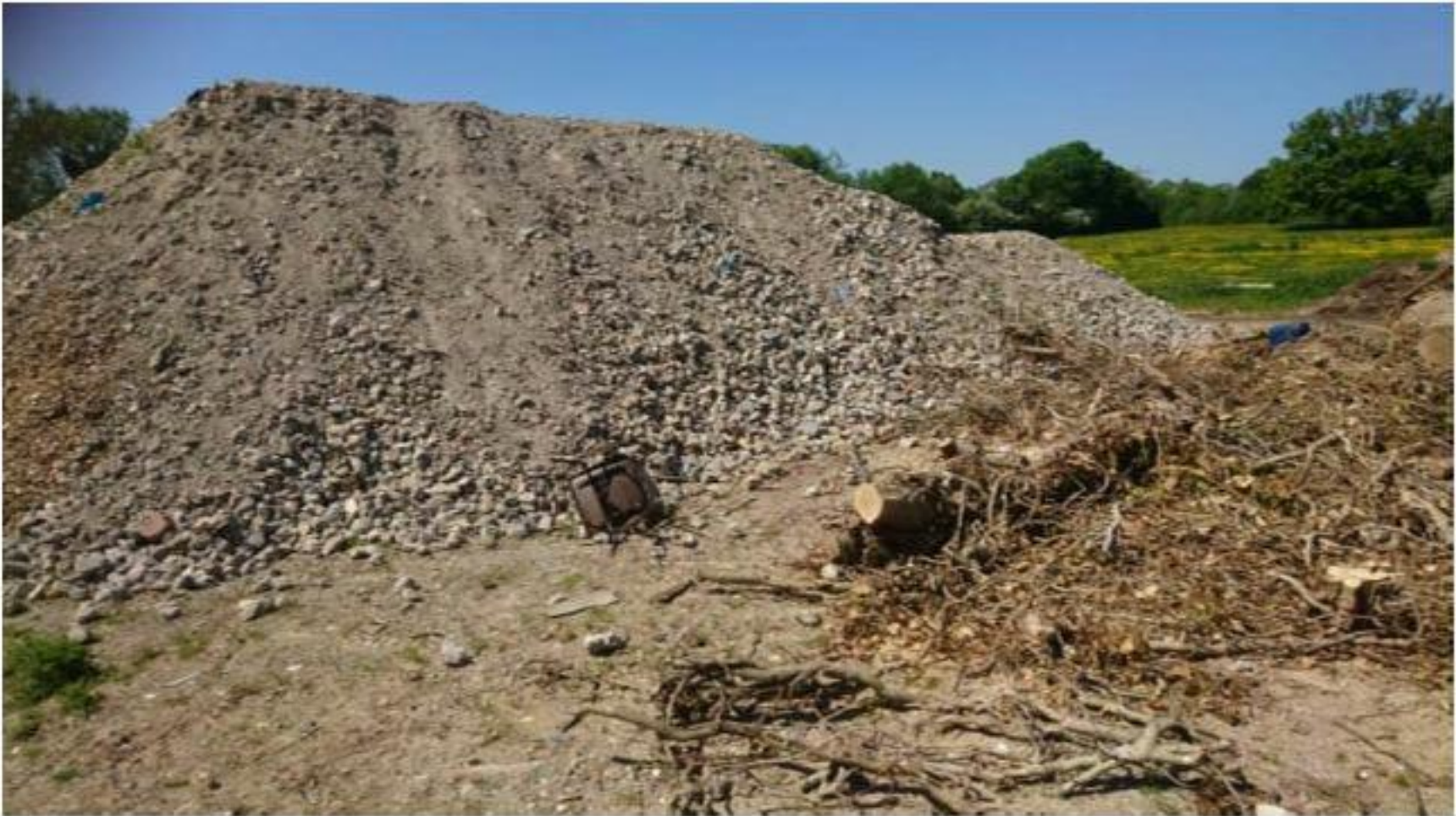
Plate 7 View of stockpiled crushed concrete material, stored in north western side of the farmyard area
