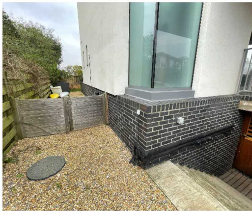
Image 03 – Access to the basement
