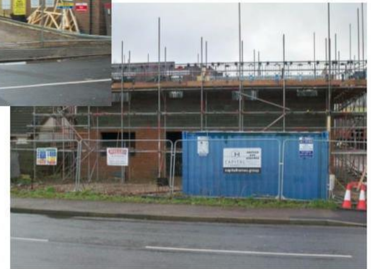
18. Current development to the rear of 160 Lovedean Lane
