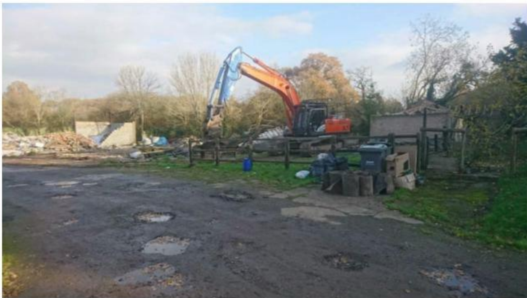
Plate 1 View north east across the former farmyard and stable area
