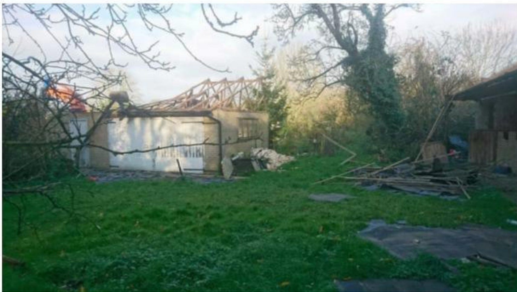
Plate 4 View of former garage building associated with the farmhouse with possible asbestos sheeting stacked adjacent to building
