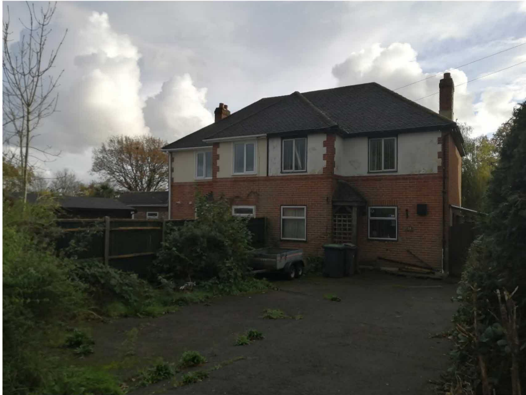
Fig. 15 - View of No. 24 Padnell Rd.
