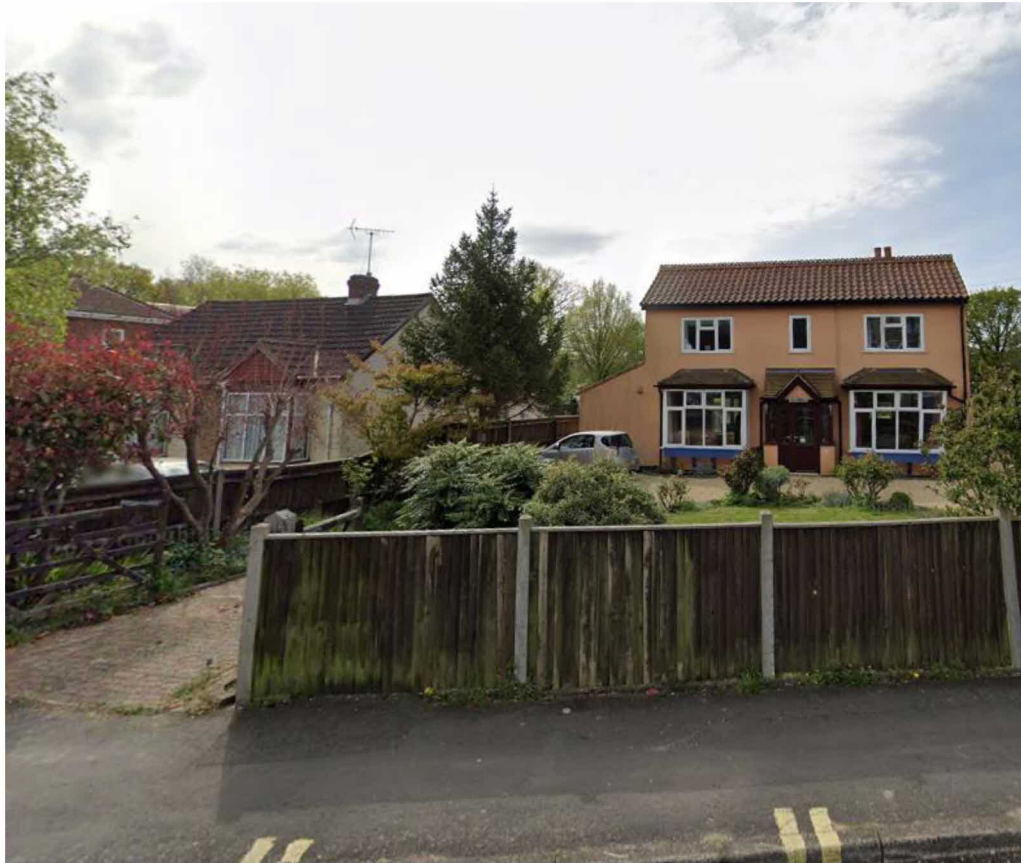
Fig. 17 - View of No. 16 Padnell Rd.
