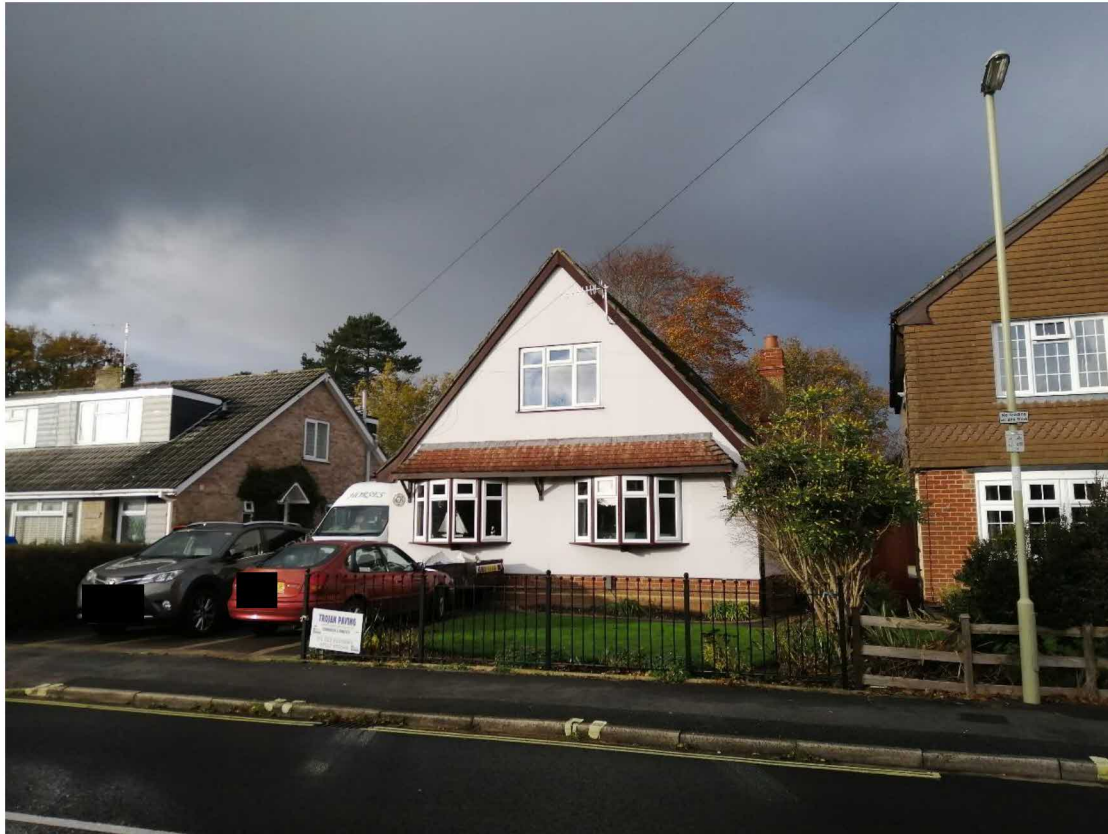
Fig. 21 - View of No. 9 Padnell Rd.
