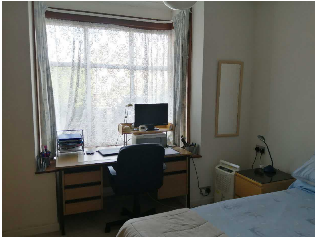
Fig. 06- One of the bedrooms affected by the works. There is too much light and not enough privacy in these street-facing bedrooms, hence the renewal of the bay windows with less glazing.
