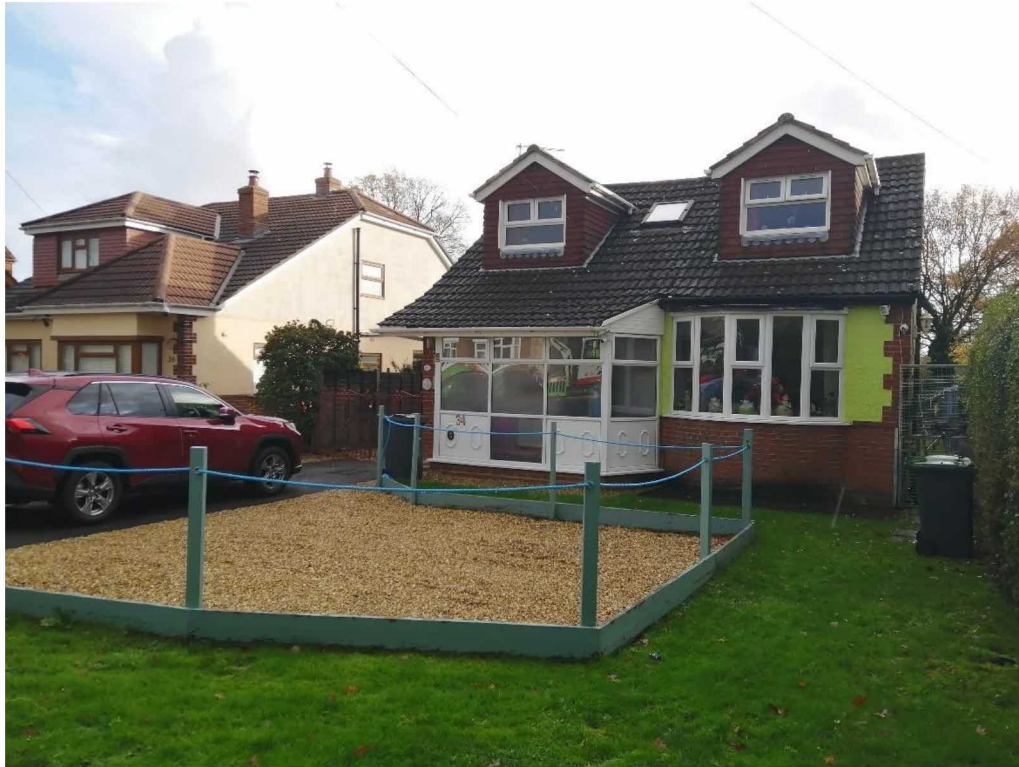
Fig. 19 - View of No. 34 Padnell Rd.
