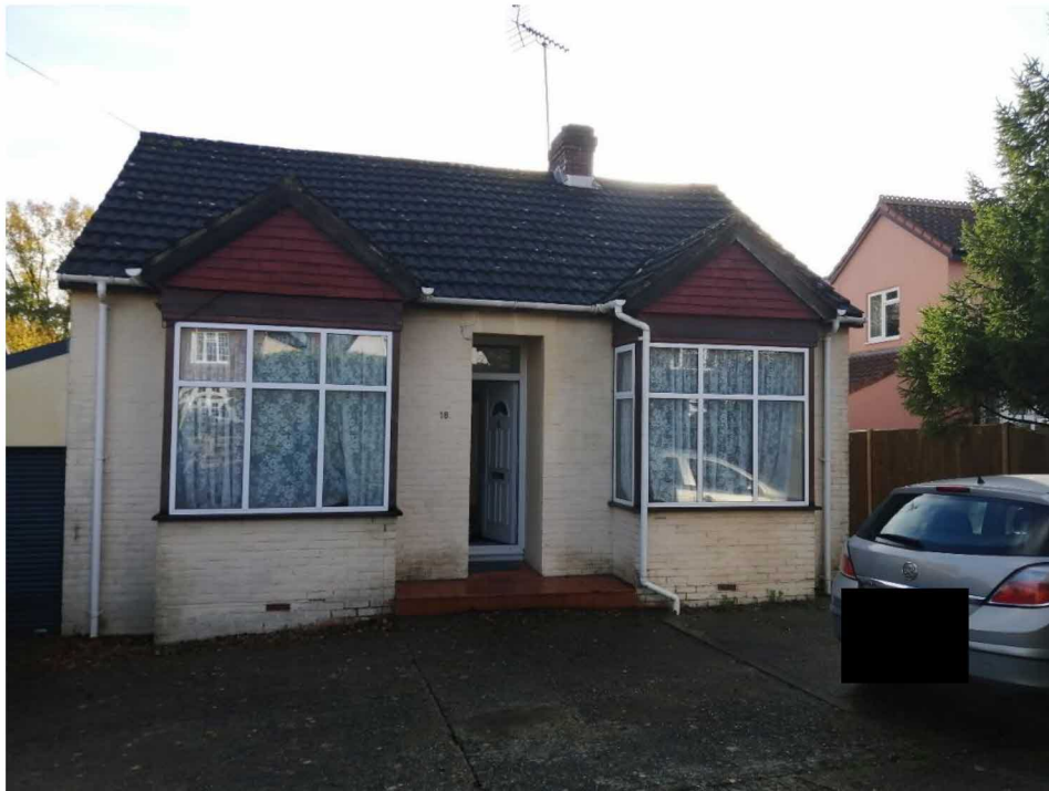
Fig.02 - Existing front of property. This will remain the same, except for the removal of the side window panels in the bay windows, and an infill porch.
