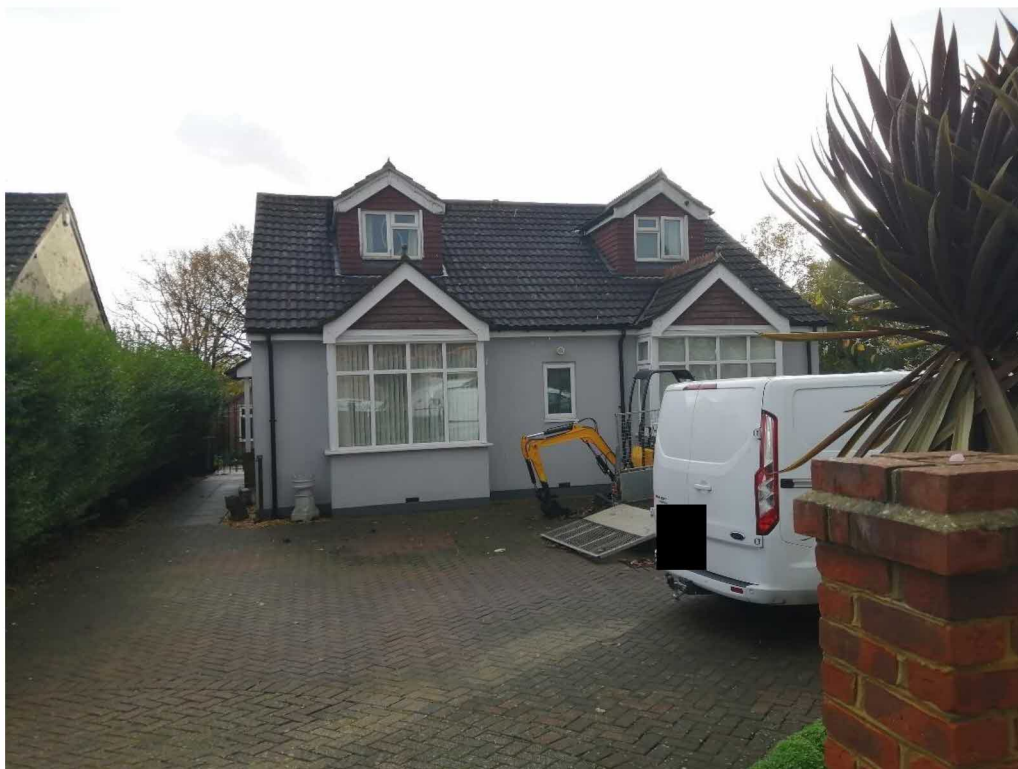
Fig. 18 - View of No. 26 Padnell Rd.
