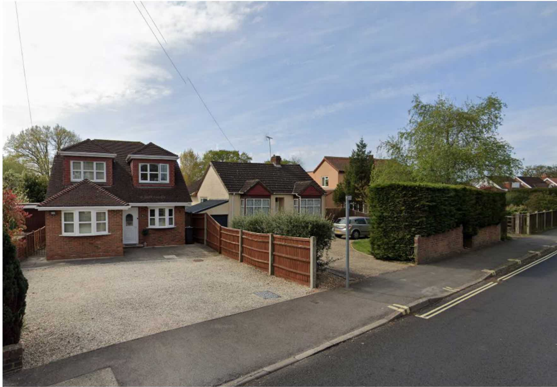
Fig. 13 - View of No. 20 and 18 Padnell Rd.
