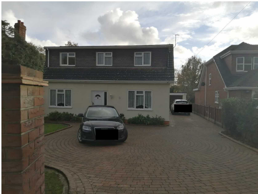
Fig. 14 - View of No. 22 Padnell Rd.
