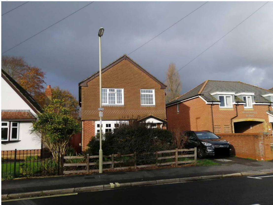
Fig. 22 - View of No. 11 Padnell Rd.
