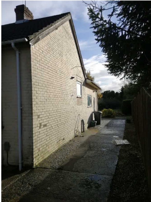
Fig.08 - Side view of house, looking from the driveway (left).
