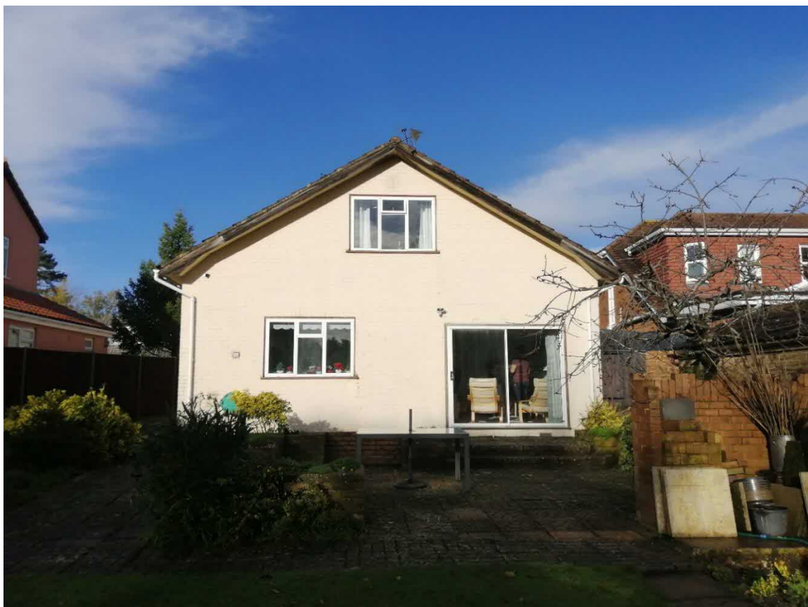
Fig. 10 - View of rear of house.
