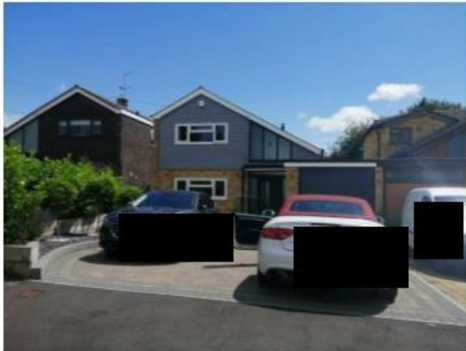
View of the existing front of the property.
