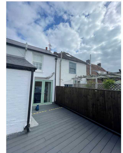
View from Existing Terrace – Looking N.E
