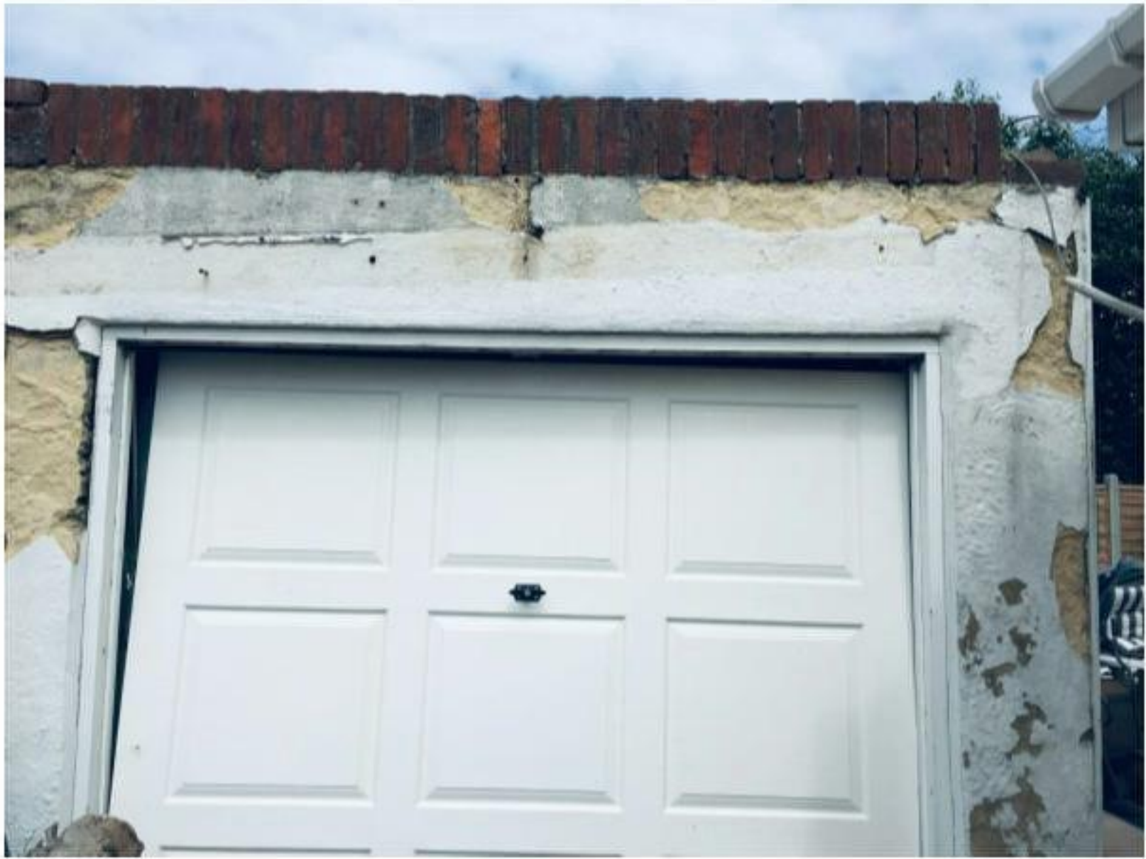
Photo 9: Front of garage
