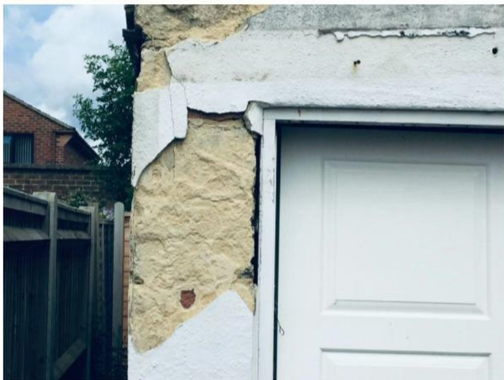
Photo 10: Side of garage
