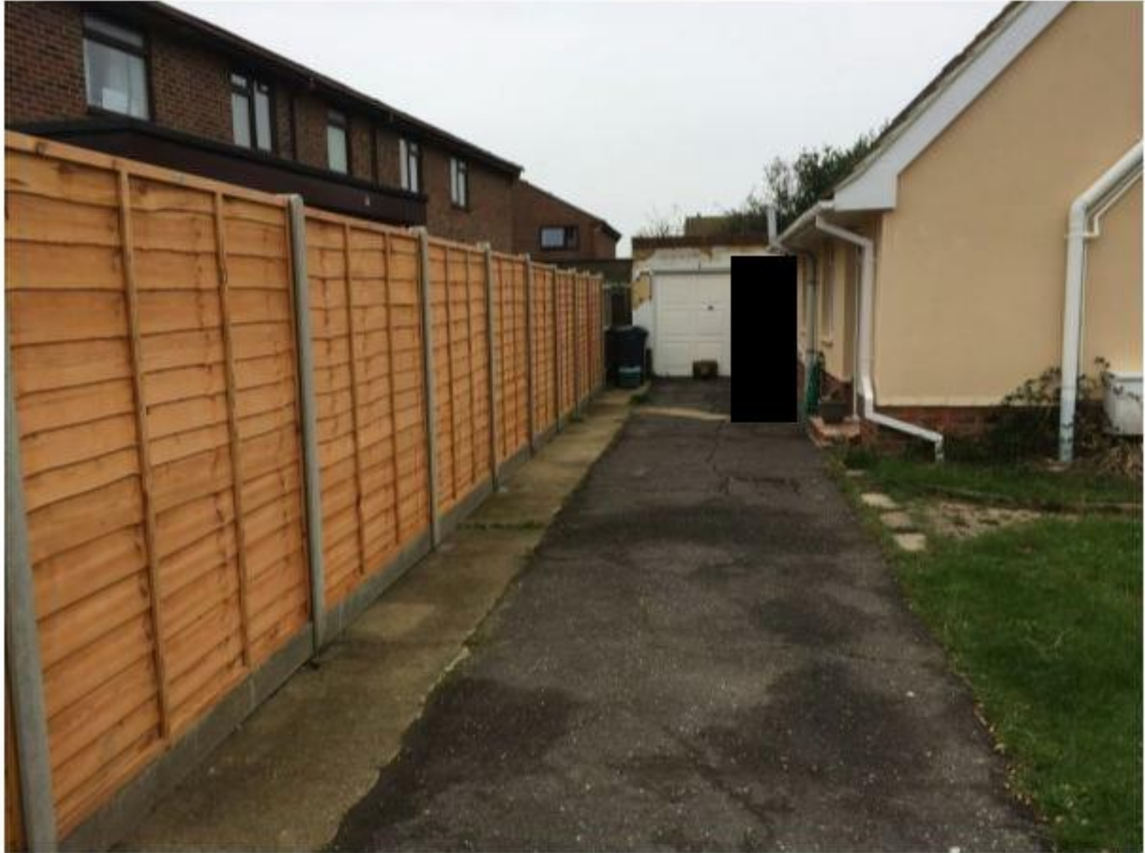
Photo 1: Front of Garage
