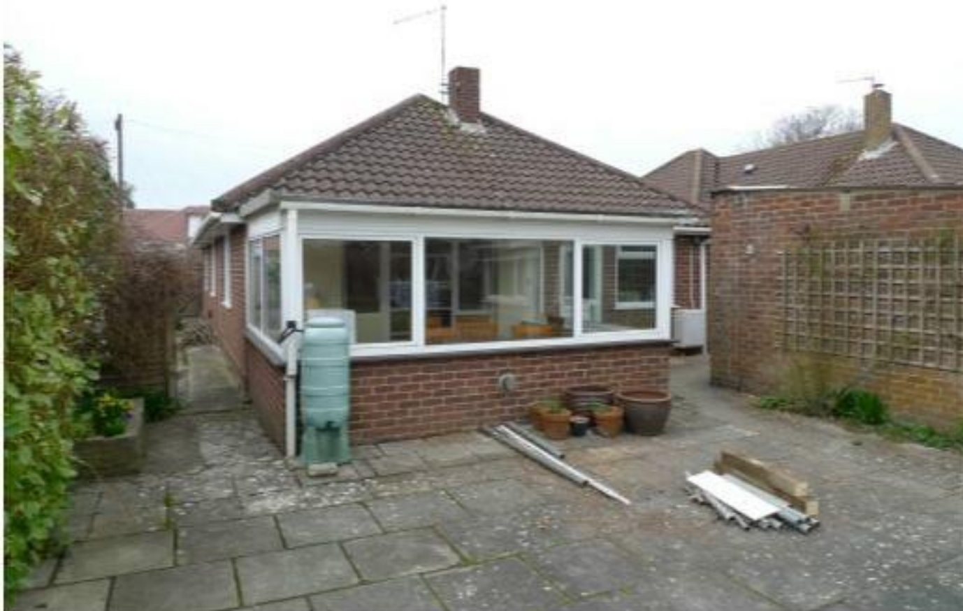
Rear elevation showing the existing extension
