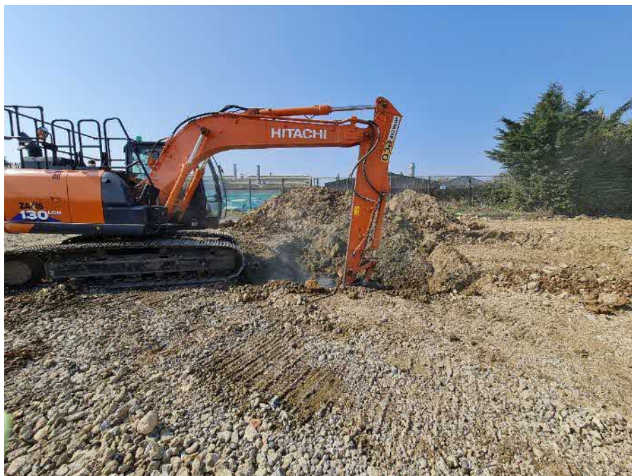
Figure 19 – Addition of E-Clay additive and inn-situ soil mixing to required depth.
