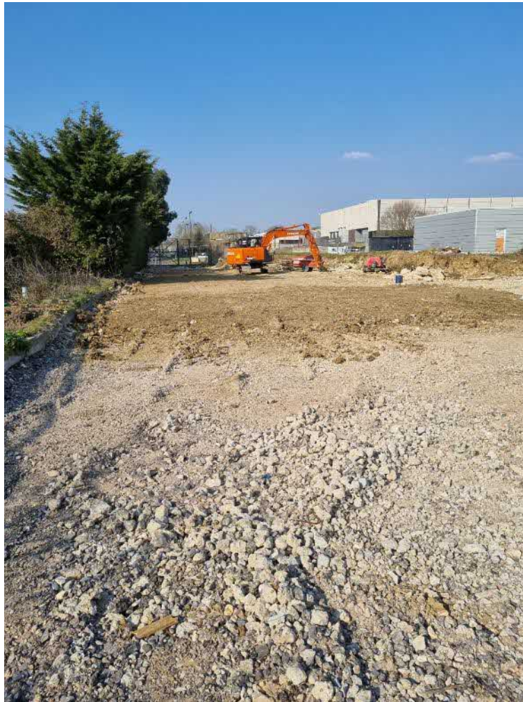
Figure 23 – Area following completion of treatment works..
