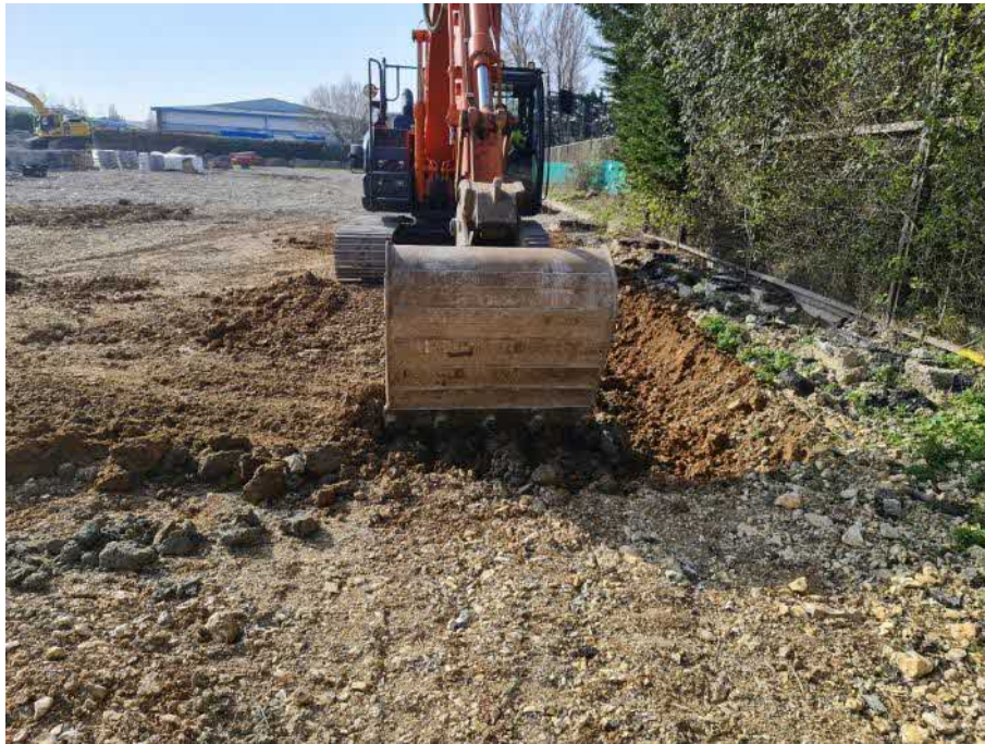
Figure 16 – Excavation of Treatment Grid Area to 1m bgl.
