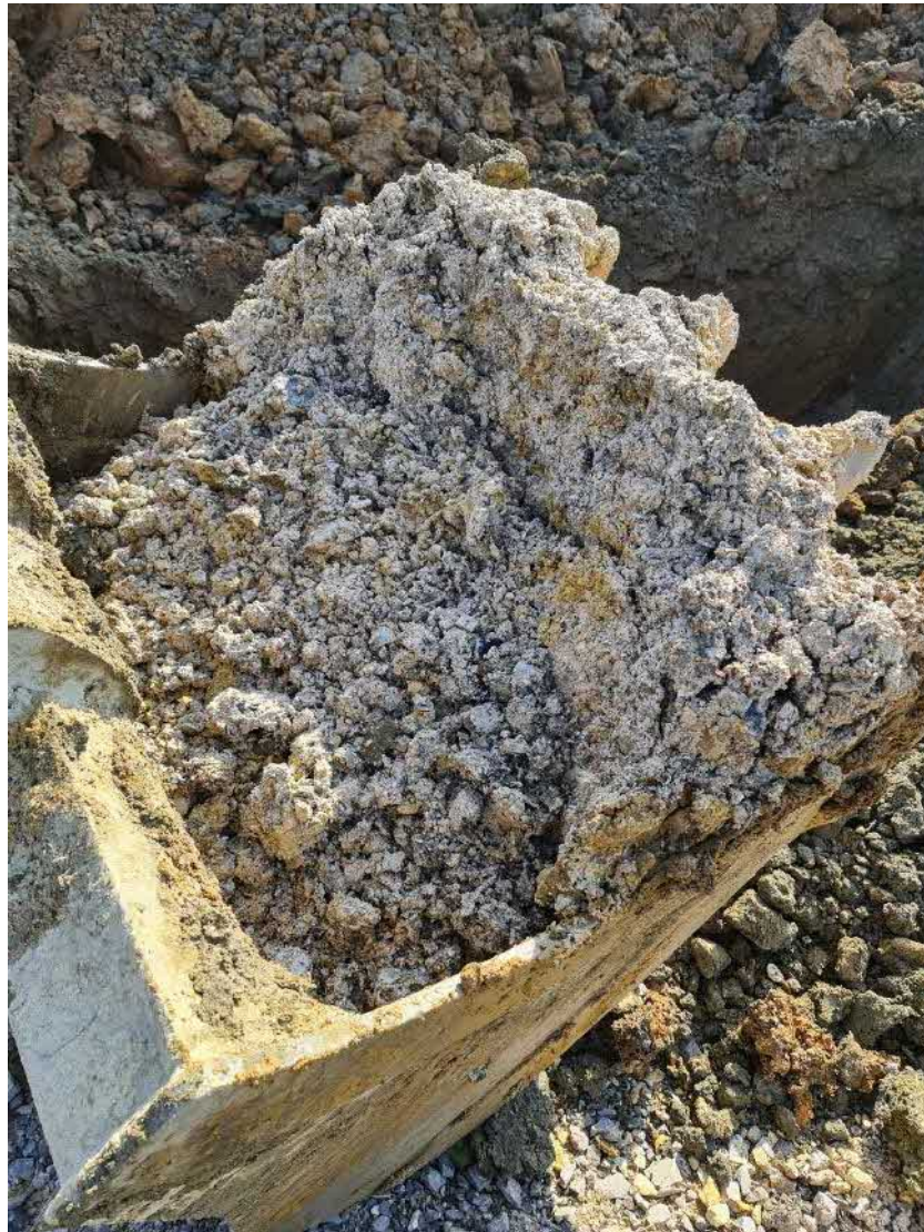
Figure 22 – “Clean” clays from base of excavations (natural in appearance, no staining, no odour & no VOC).
