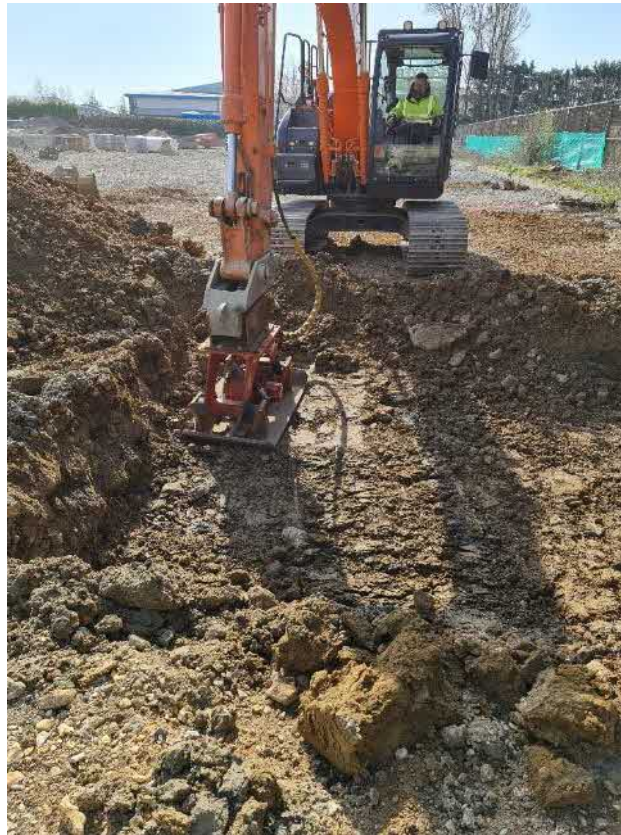
Figure 20 – Reinstatement of treatment Grid area post treatment.
