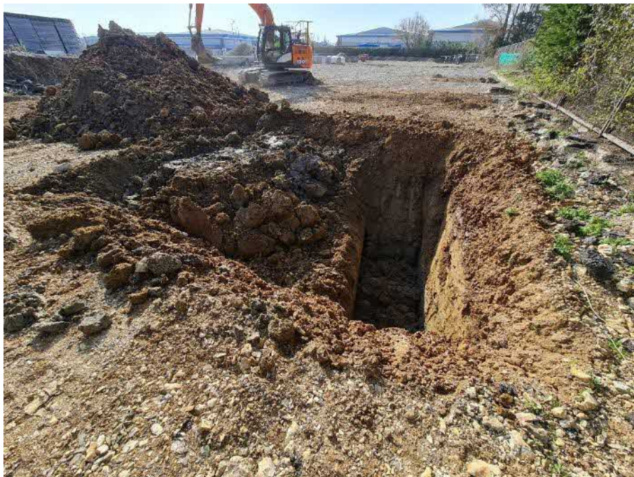
Figure 17 – Fully excavated Treatment Grid (Half) Section for Treatment.
