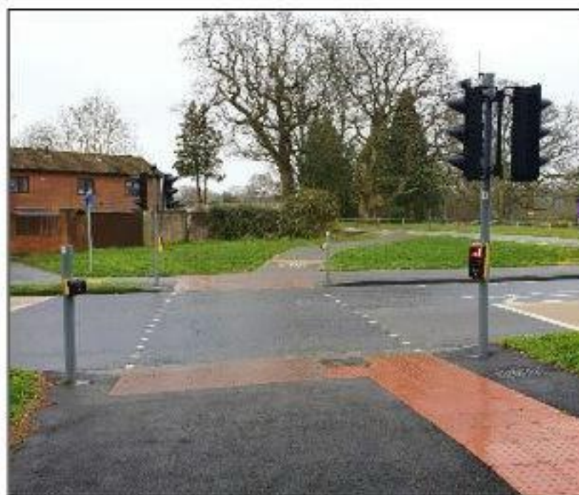
Photograph 4. Toucan crossing facility
