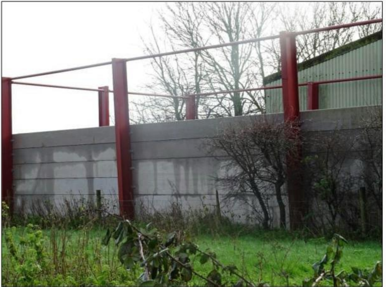
Close up view, from North Farmhouse boundary.
