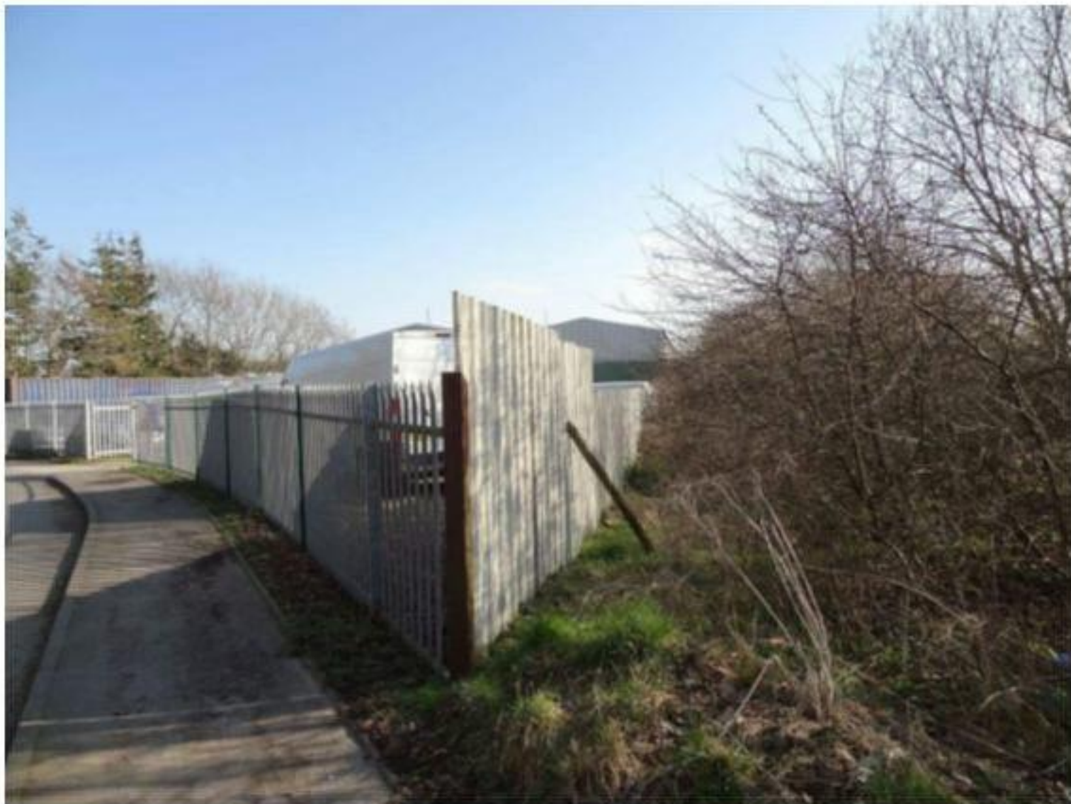
Photo 4 – View from footpath in Mill Rythe Lane along the south-west boundary fence..
