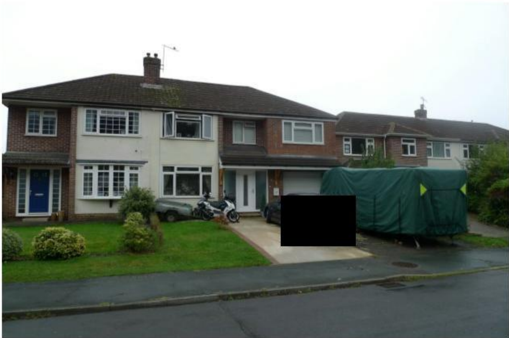
The front elevations of 40 and 42 Burnside showing the ridge line to number 40
