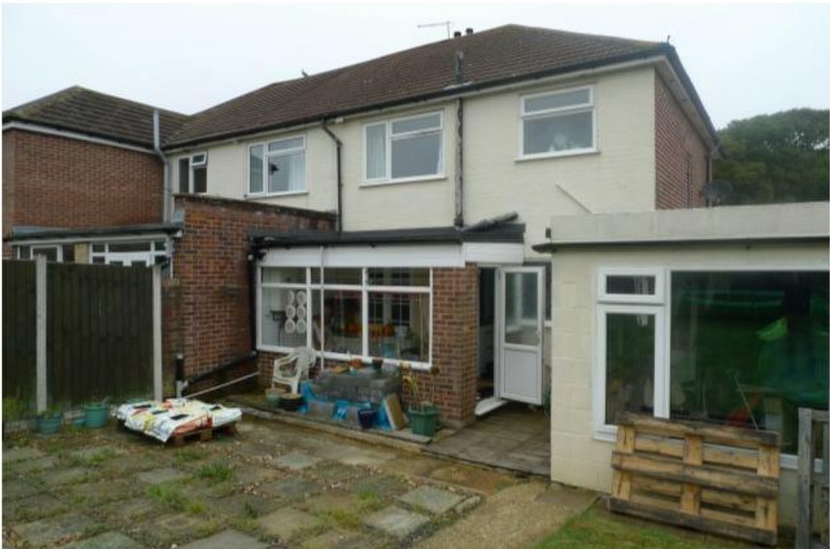
The rear elevation of 42 Burnside – camera faces north west.
