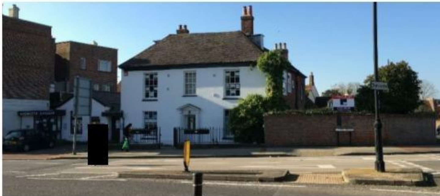
Plate 6: 6 North Street, principal east elevation.
