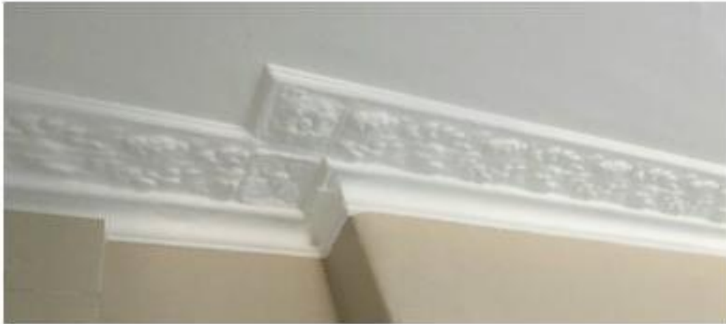
Plate 29: Decorative cornice, Room 3a.
