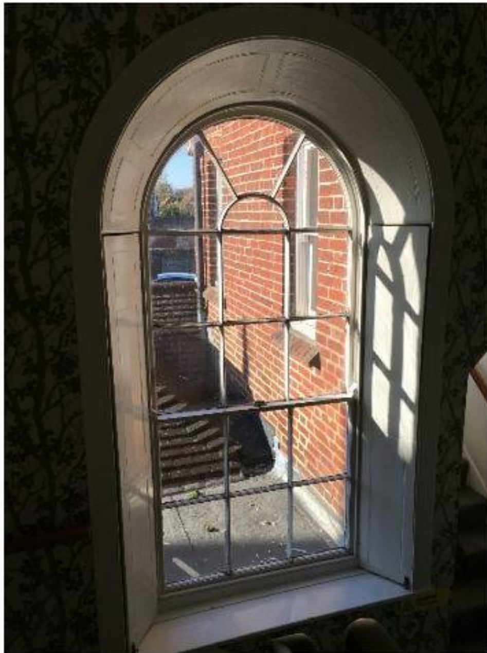
Plate 32: Window above the main staircase (Room 10).
