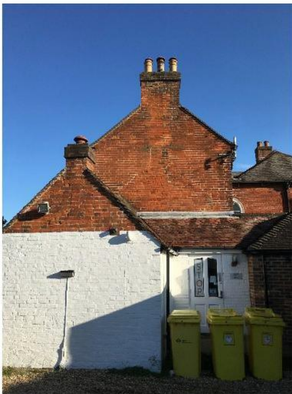
Plate 21: East-facing view to the rear (west) elevation of the north range.
