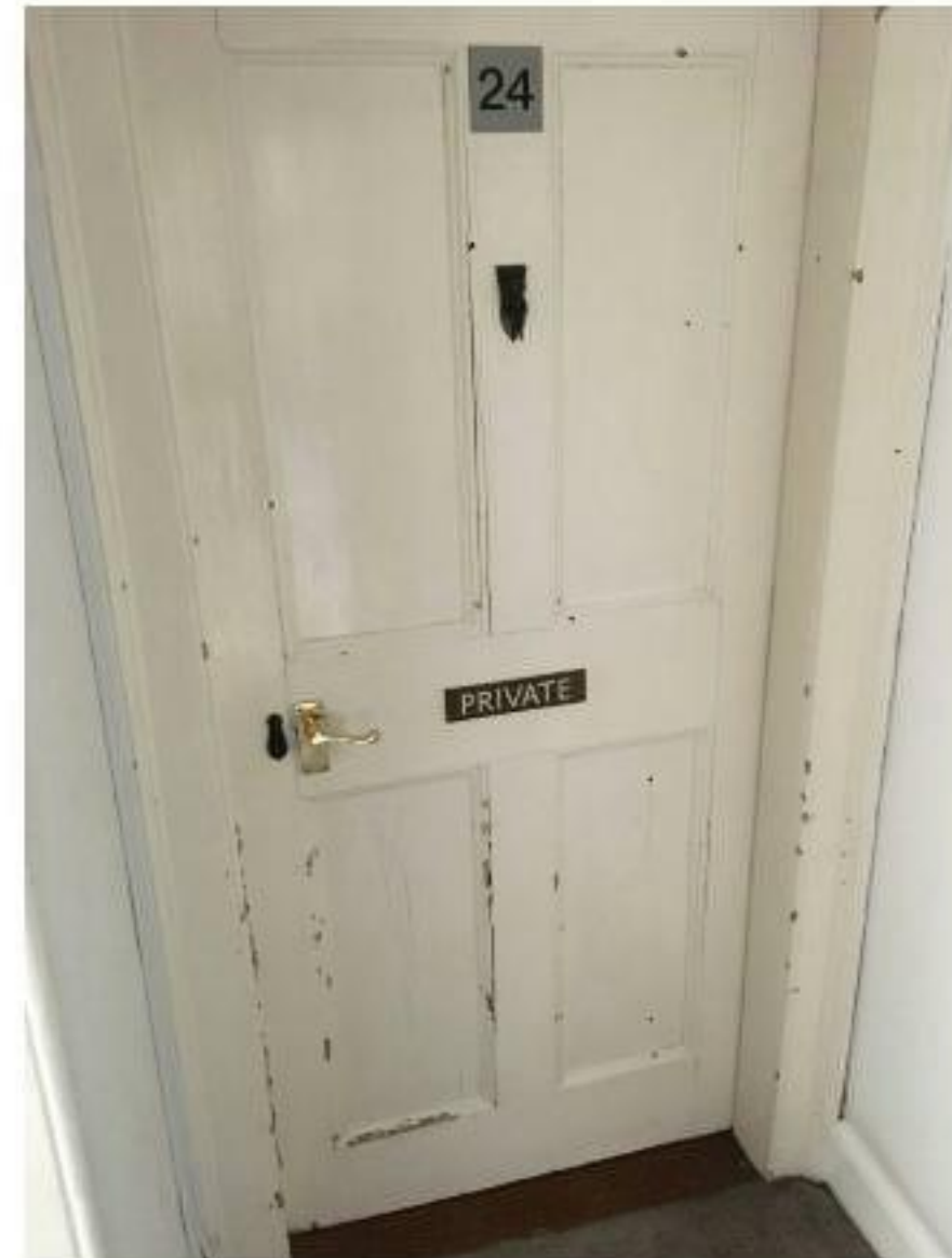
Plate 31: Door to Room 15 (labelled 24) from Room 11.
