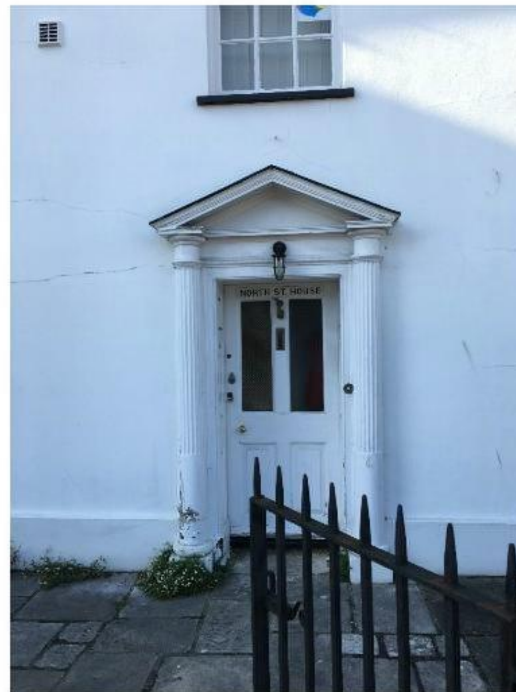
Plate 16: Detail of pedimented doorway.
