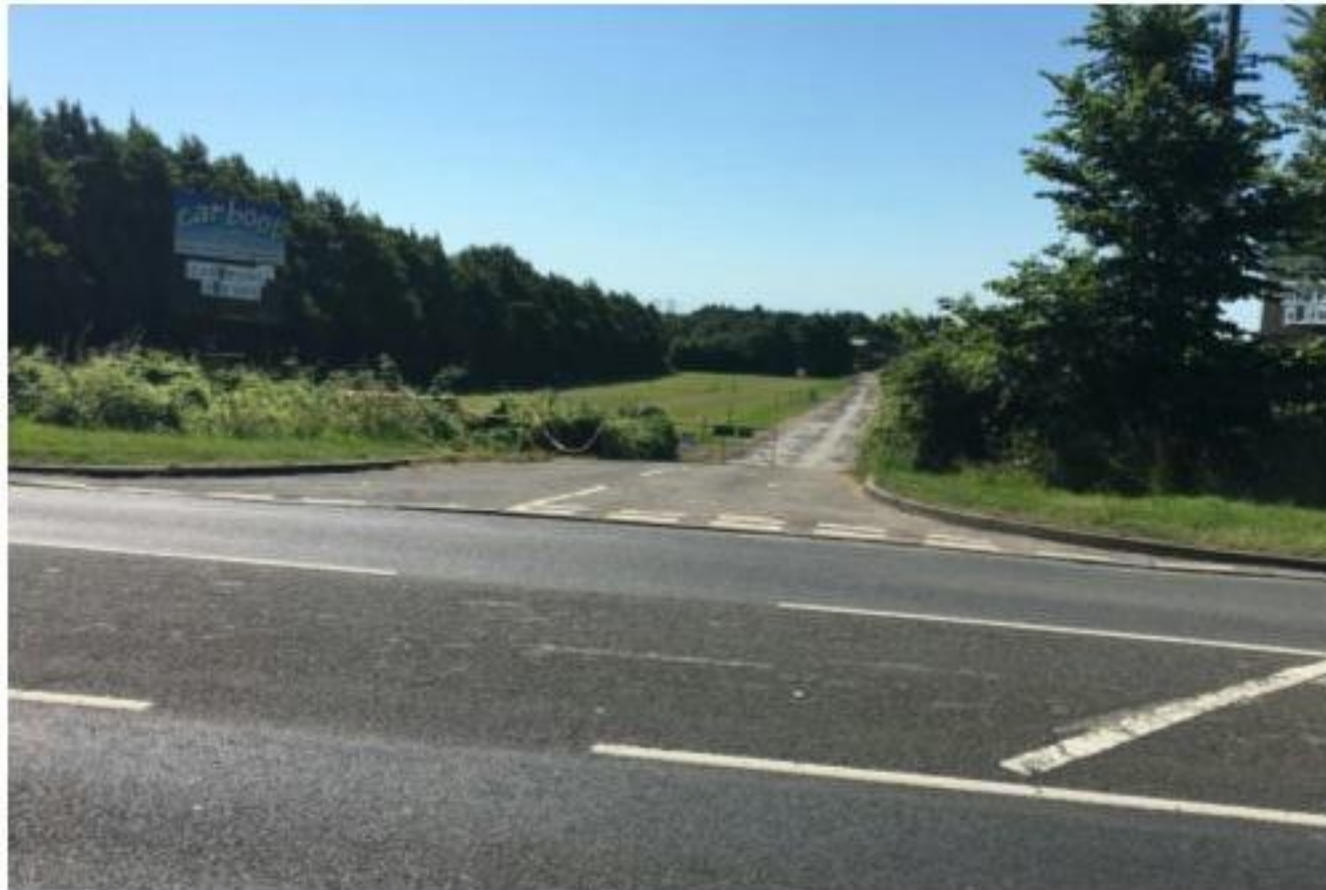
Photograph 1: Existing Site Access
