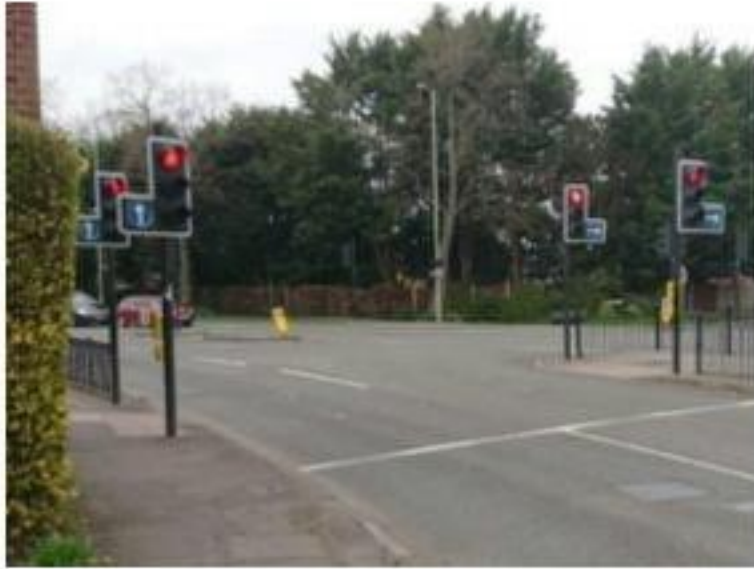
Photograph 13: Signalised junction of Bedhampton Road/Hulbert Road
