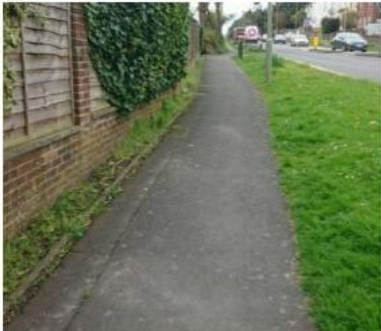
Photograph 17: Pedestrian footway along southern side of Bedhampton Road
