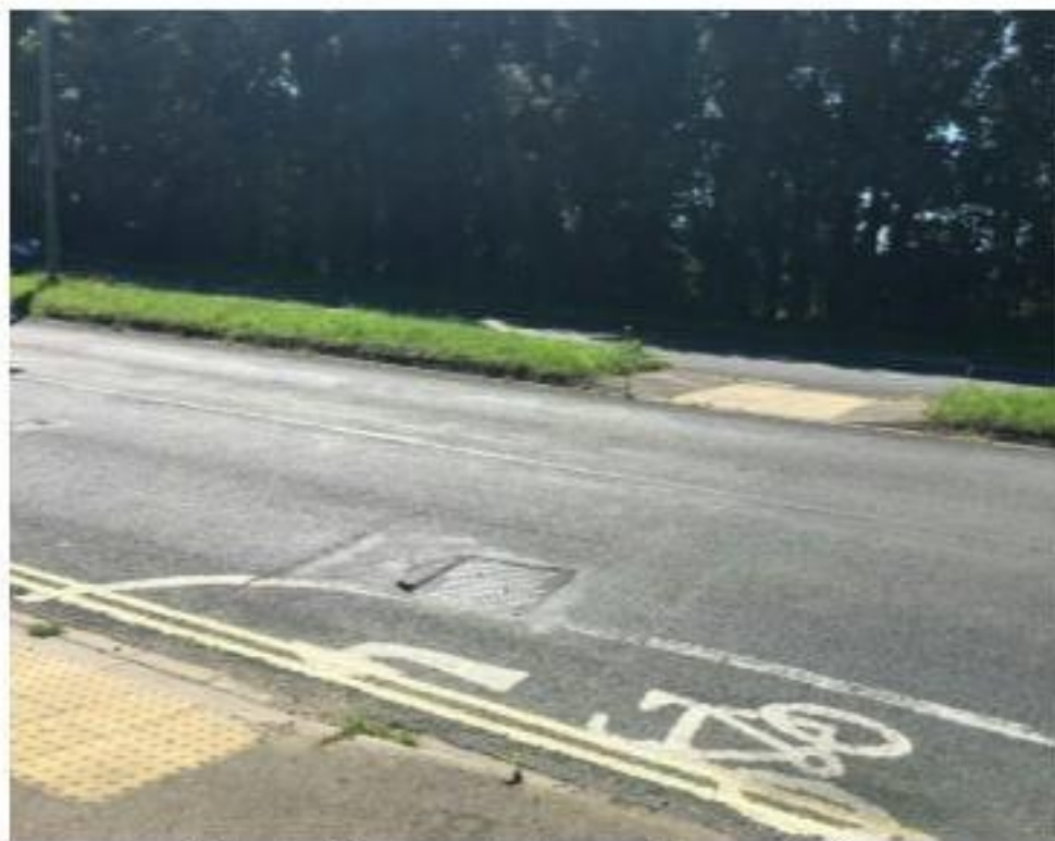
Photograph 9: Existing Pedestrian Crossing facilities
