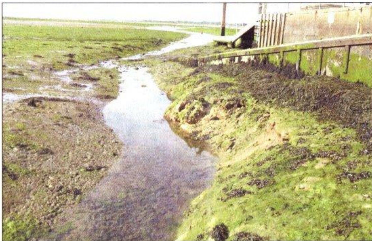
Photo 3. Existing channel from the foreshore to the east
