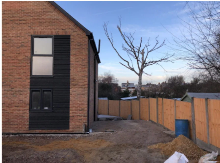
Fig.3: View looking West to location of the proposal. The dead tree in background is to be removed as part of original planning approval.
