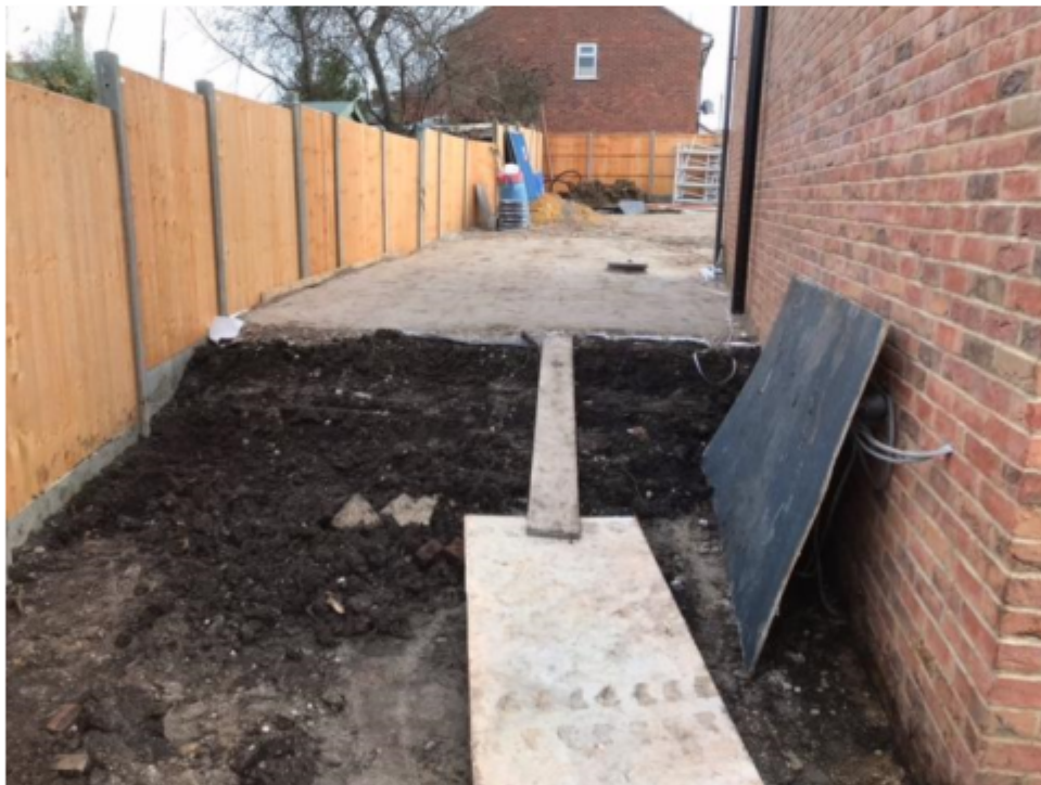
Fig.2: Image looking east showing proposed location of new office/studio. Neighbouring property 1B can be seen in background.
