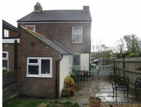
Fig 2. View of the rear of the property
