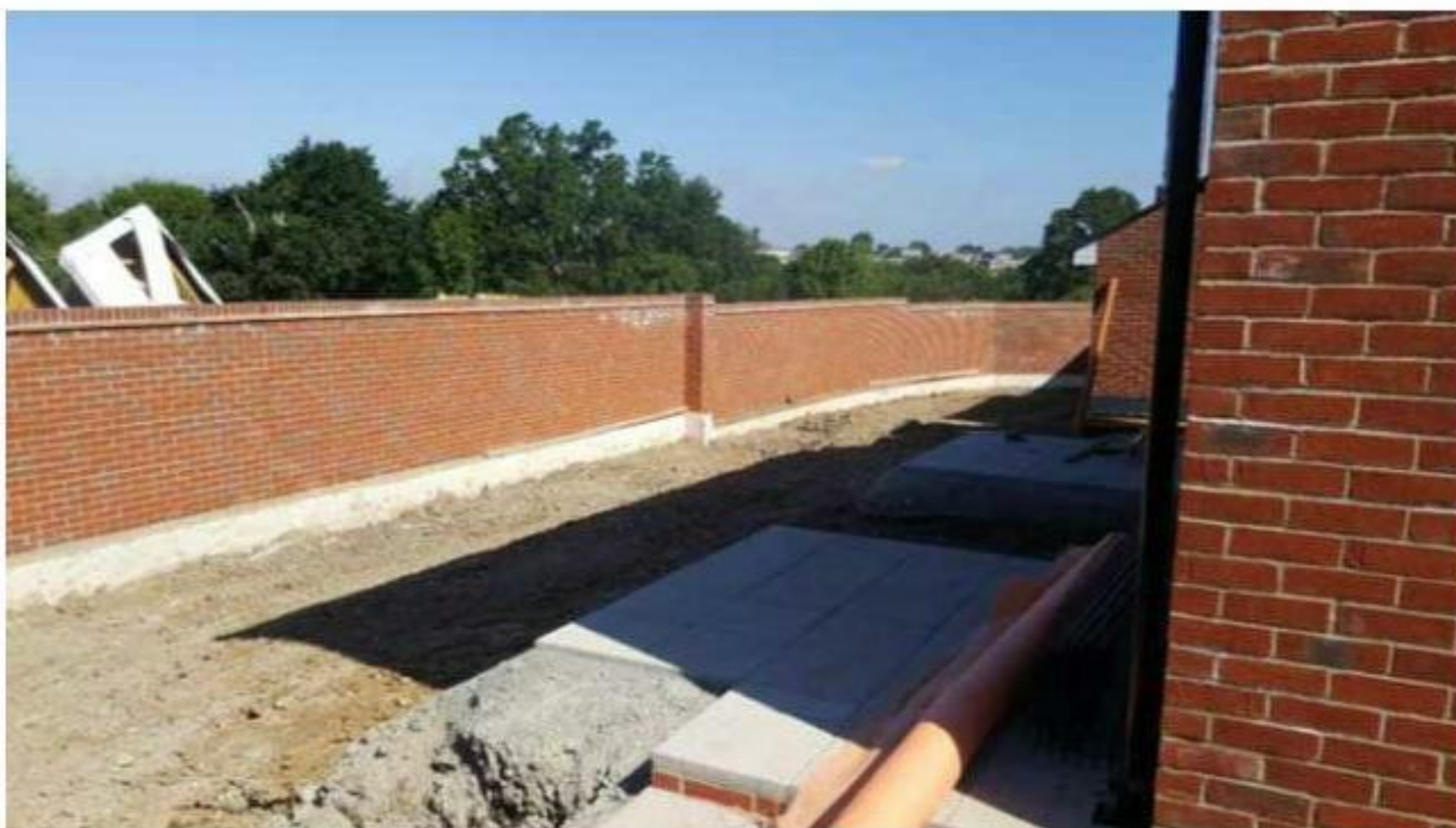
Plate 1 Plots 13-16 Gardens prior to placement of membrane, geogrid and soil cover
