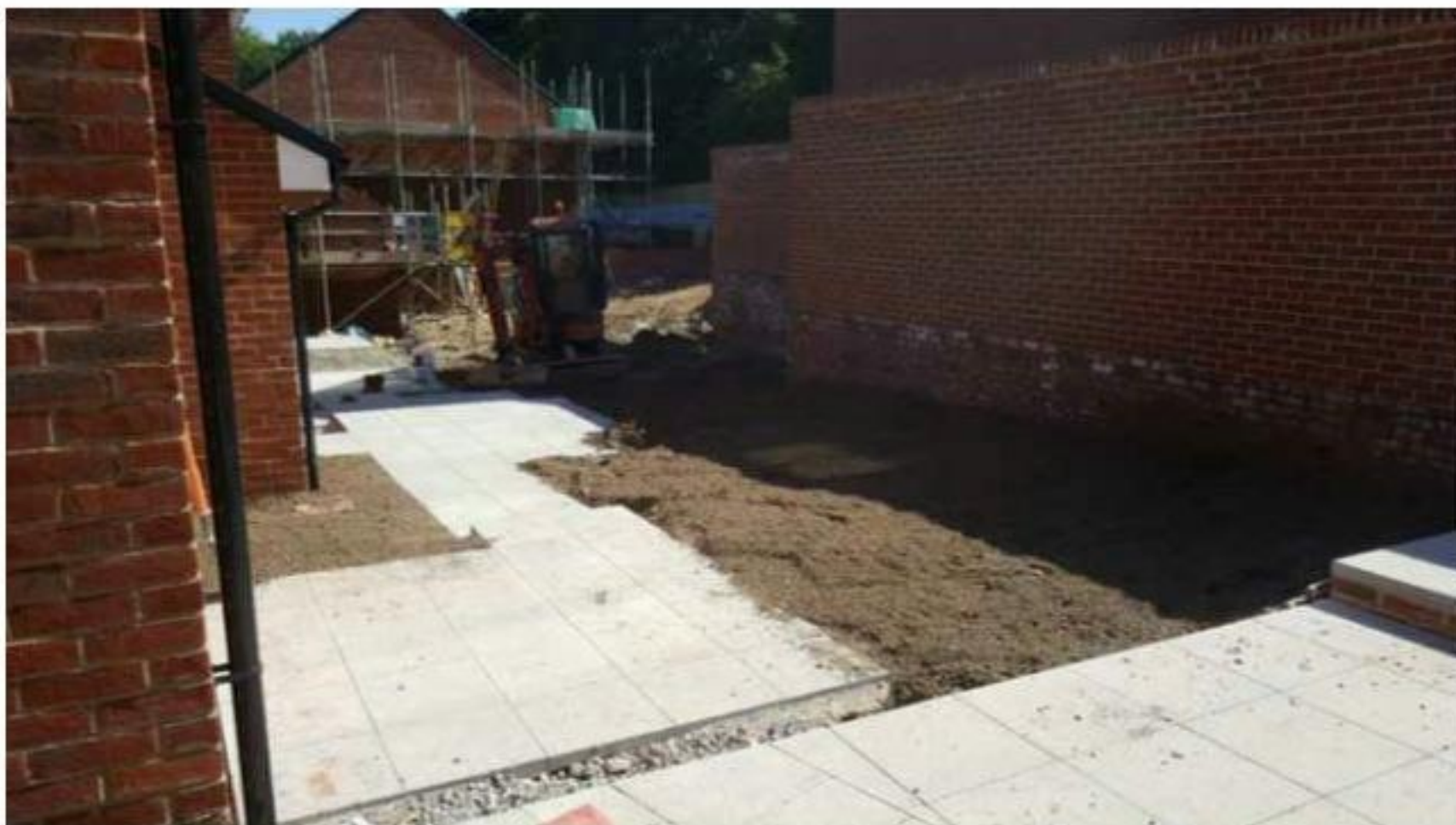
Plate 3 Plots 25-27 Topsoil being placed
