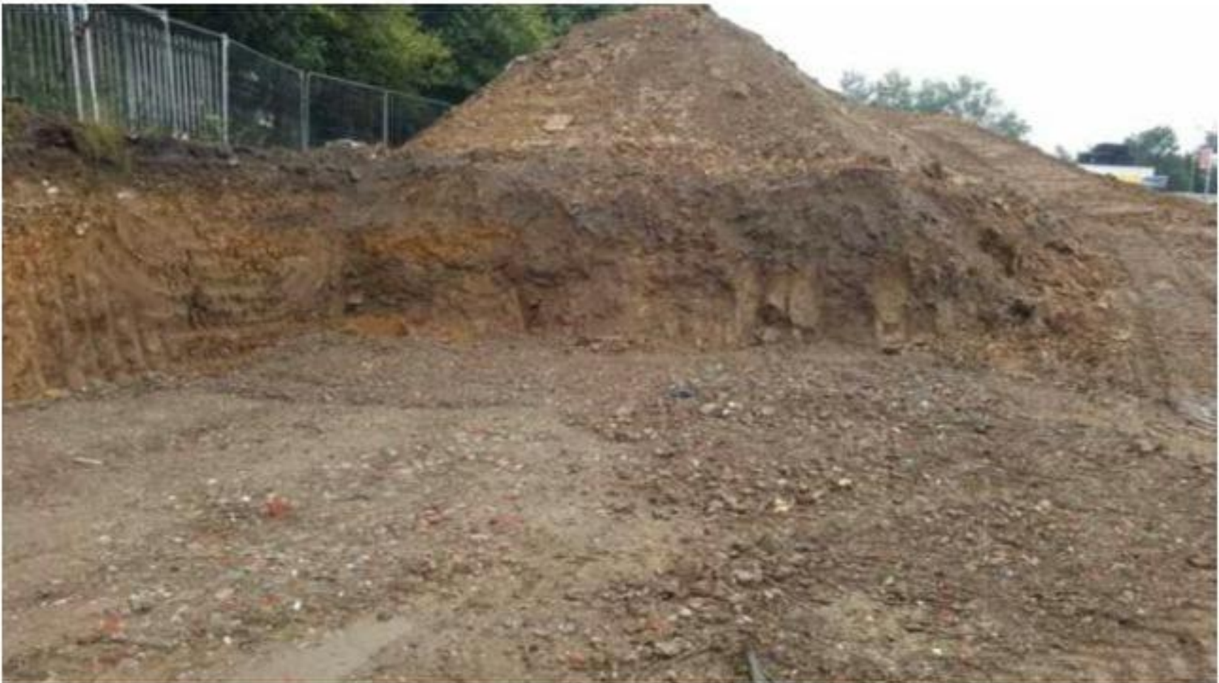
Plate 6 Reduced dig level change between Plot 30 and Plot 29 (piling mat placed in base of reduced dig)
