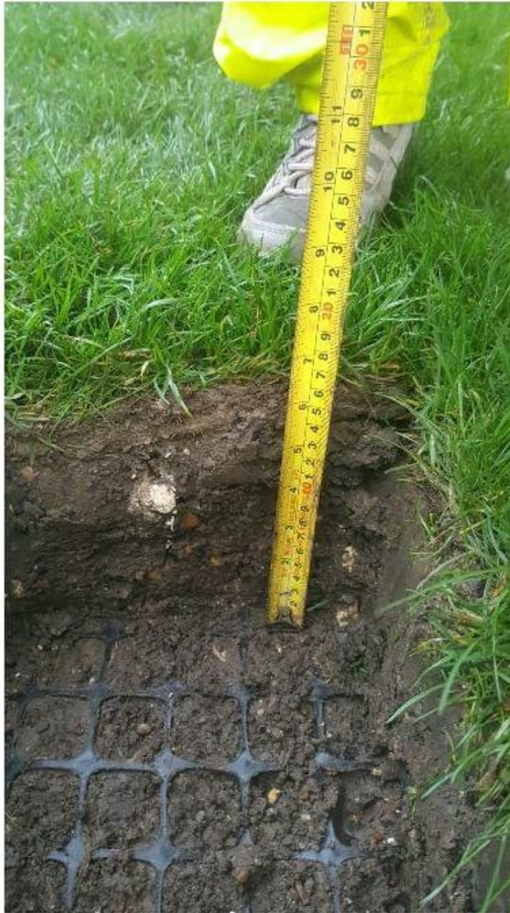
Plate 10 Plot 1-6 Pit between flats and railway cutting boundary
