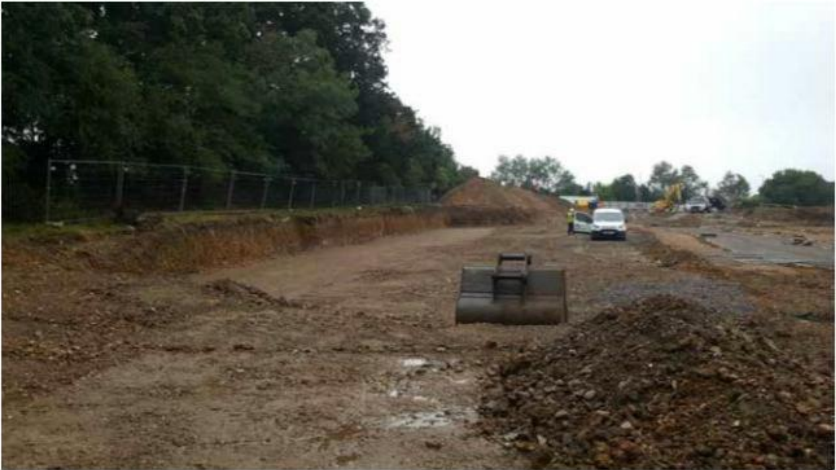
Plate 5 Plot 37 looking to Plot 30 reduced dig prior to retaining wall installation and house construction
