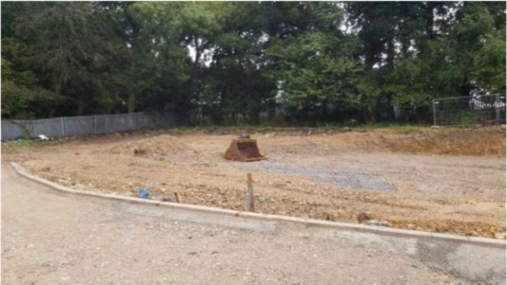
Plate 7 Reduced dig in rear of Plot 37 exposed natural soils
