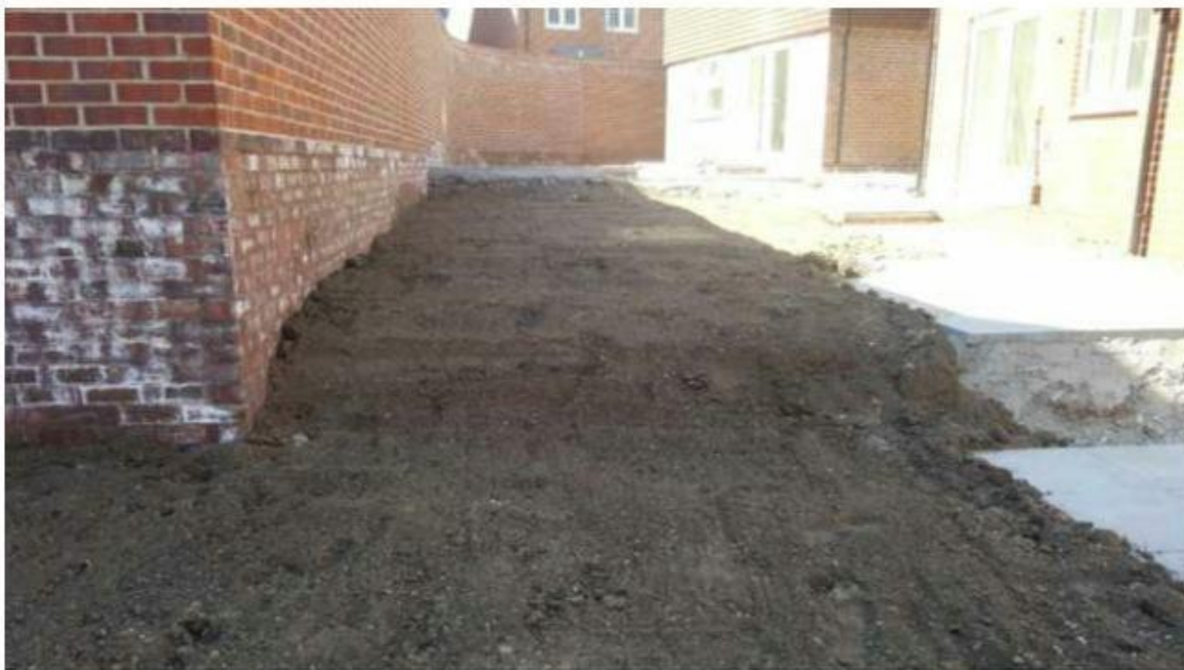
Plate 4 Plot 27 to 24 Topsoil placed
