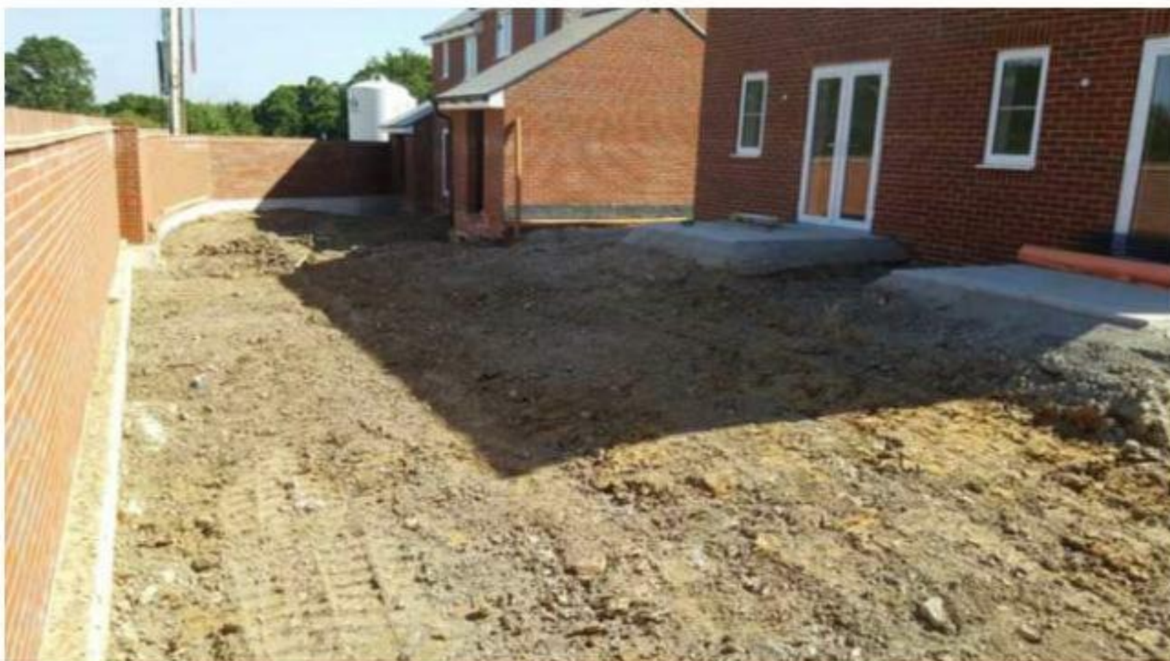
Plate 2 Plots 13-16 exposed soil formation prior to membrane, geogrid and soil cover placement
