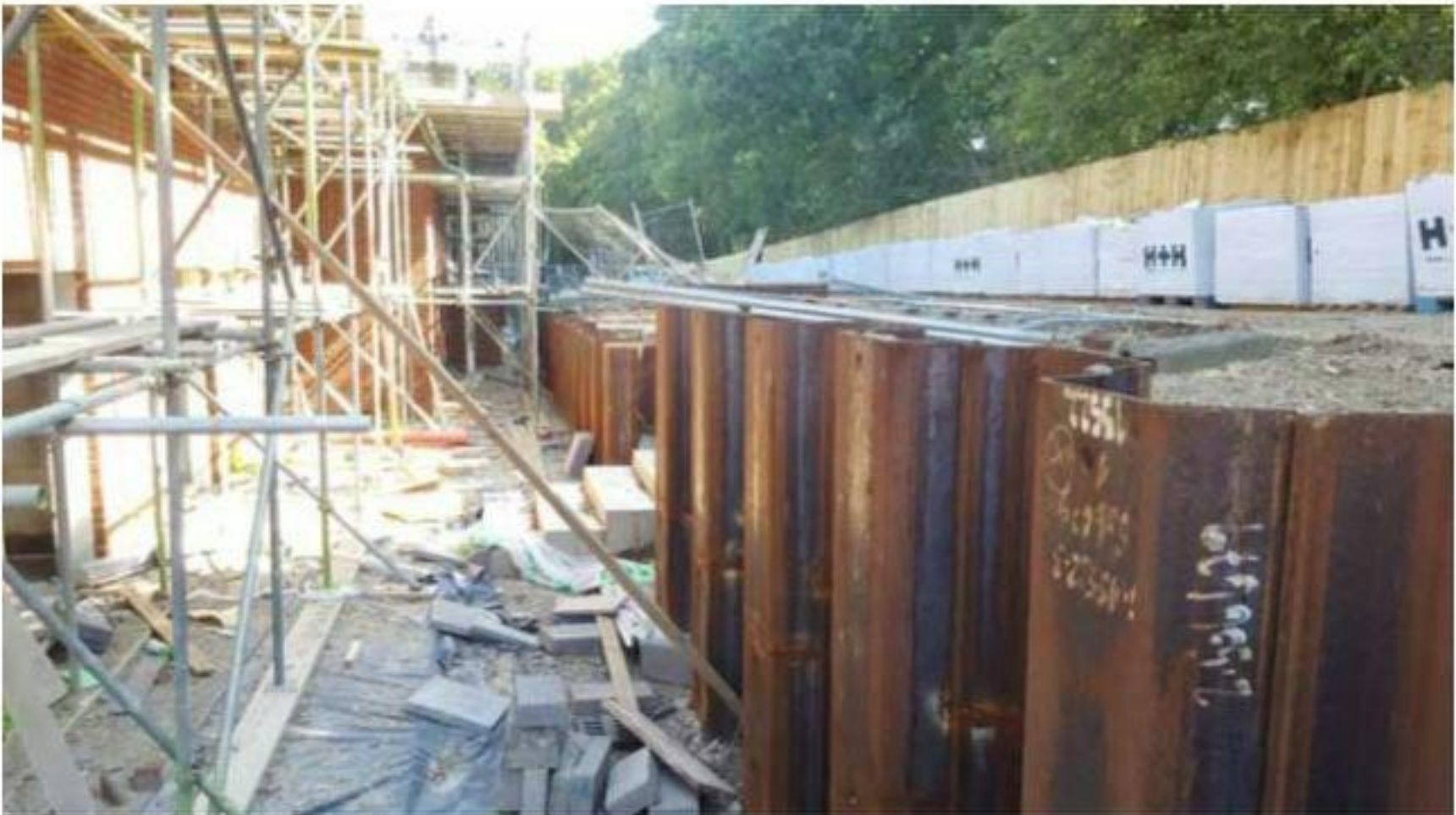
Plate 8 Sheet pile retaining wall looking from Plot 30 towards Plot 37
