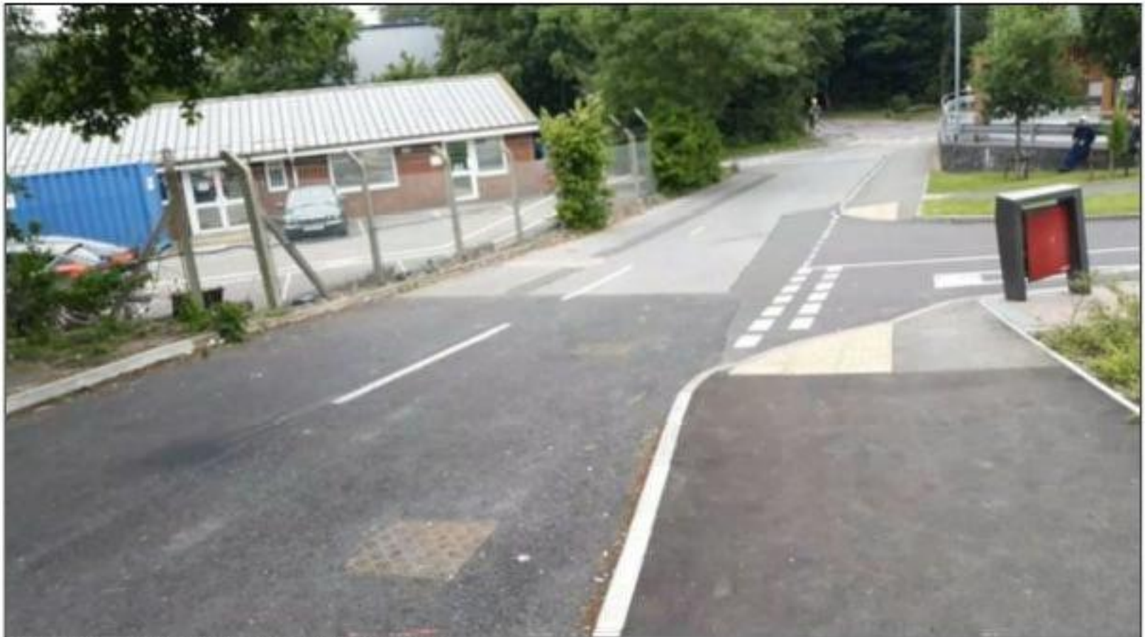
Figure 2.8 – View north along Larchwood Avenue
