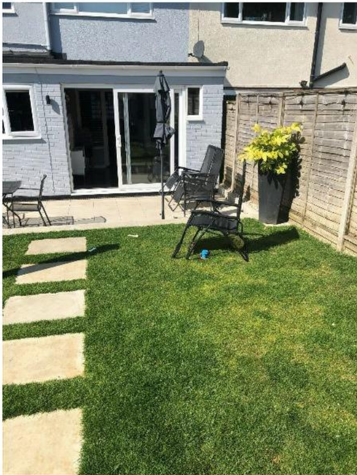
Photo 6: Rear of house
