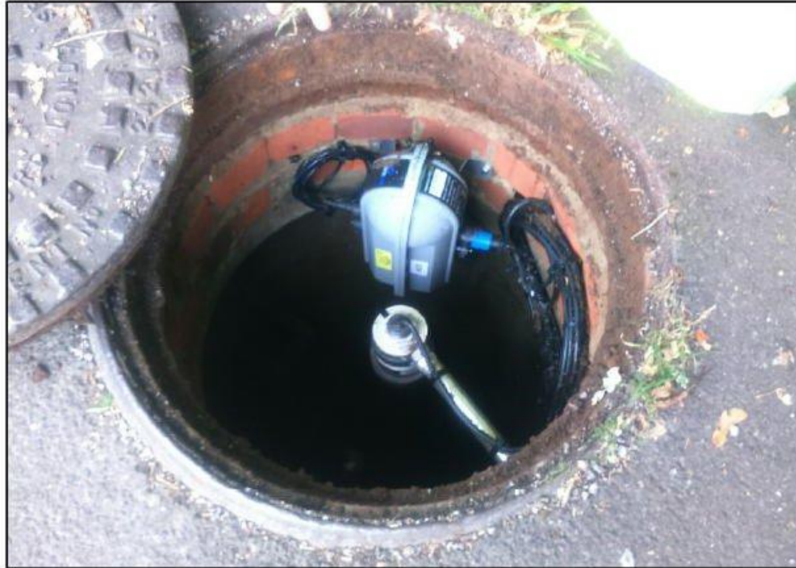
Figure 8: Photo of Southern Water Manhole 0801
