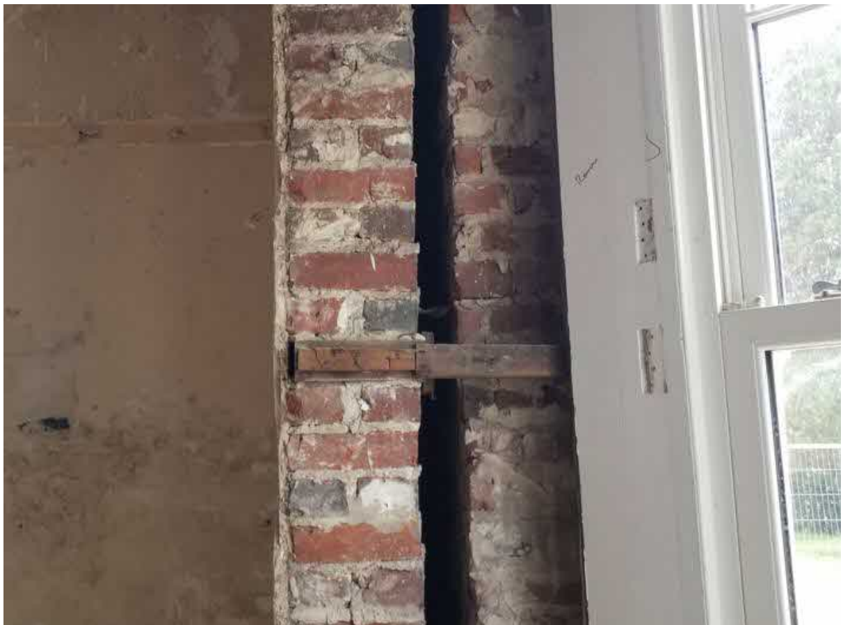
Photo 15 (External Wall structure)
