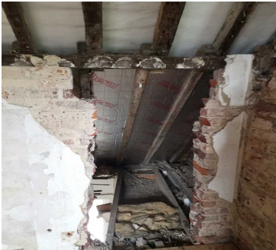
Photo 18 (Supporting wall removed)
