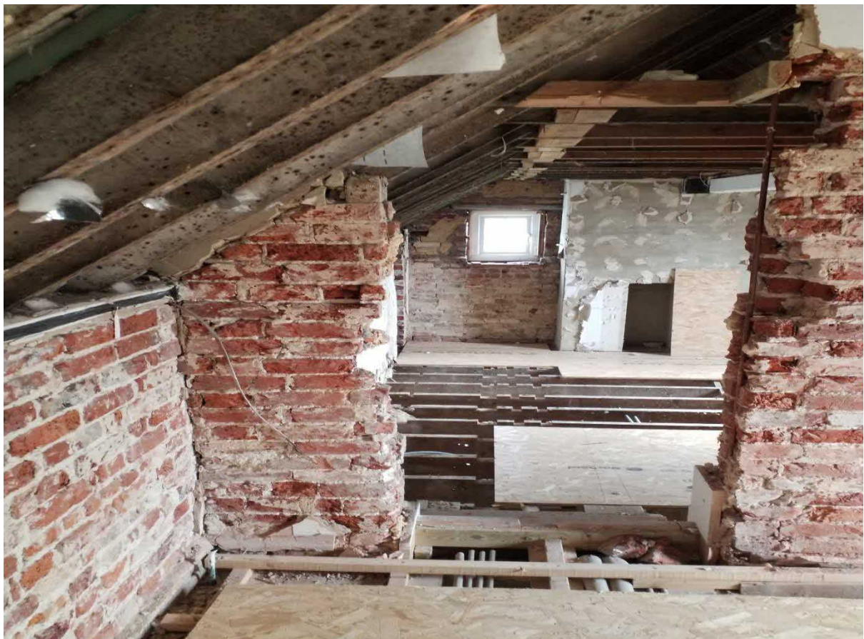
Photo 4 (Roof structure changes)
