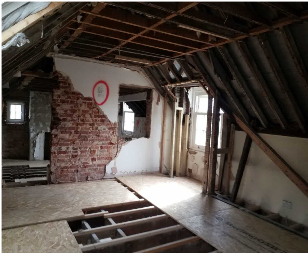
Photo 23 (Alterations to roof structure)
