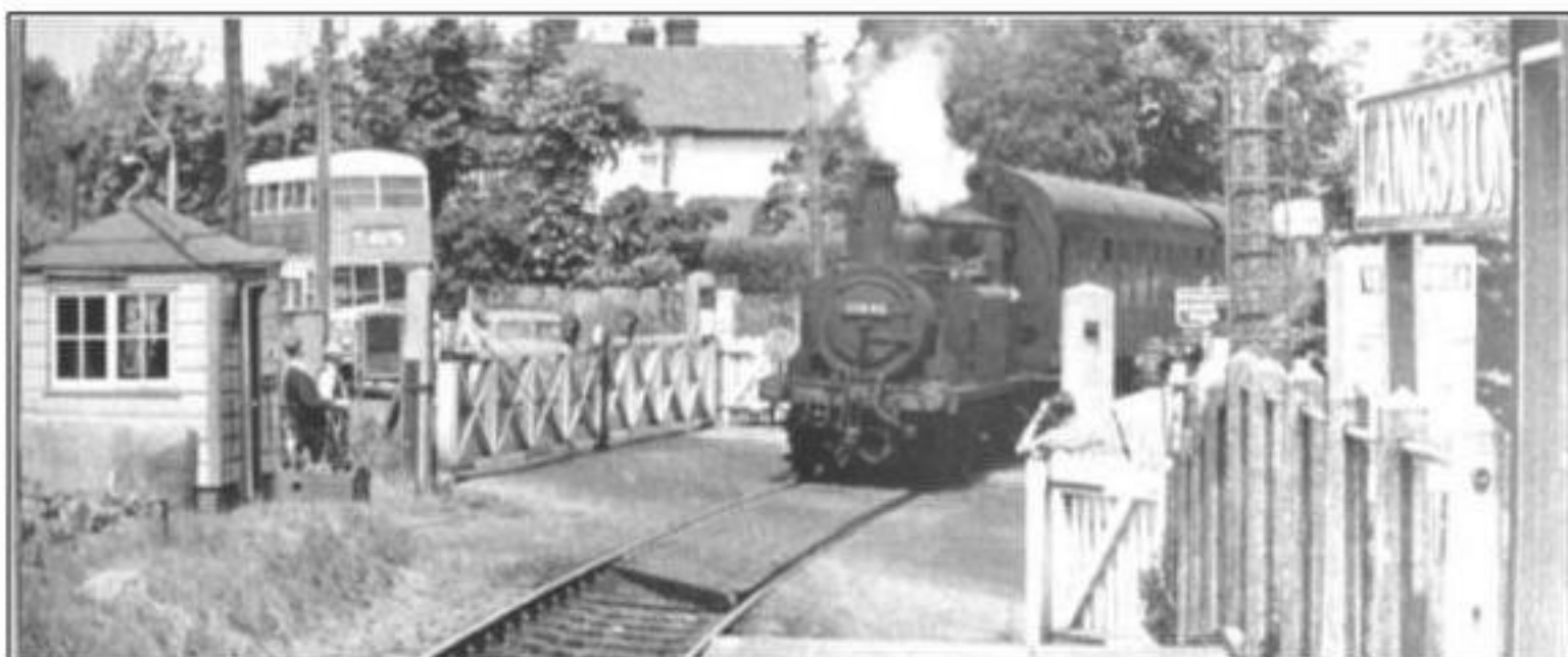
Figure 16: Langstone Level Crossing (Griffiths, G, n.d)
