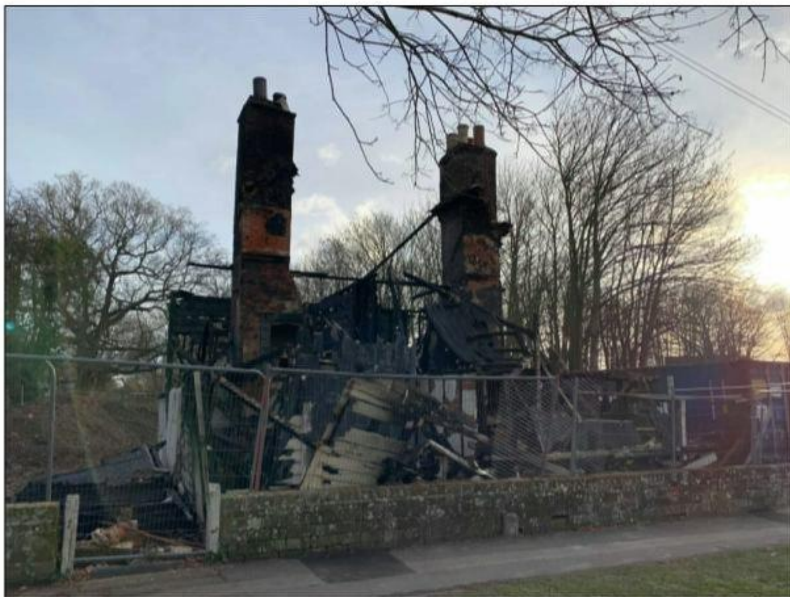
Figure 22: The cottages after the devastating fire (Jan, 2019)
