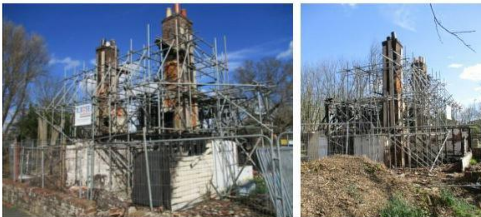
Figure 4 & 5 : Structural Scaffolding (March 2019)
