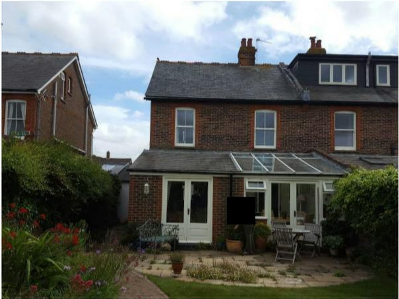
Photo 10: Rear of property where extension would be
