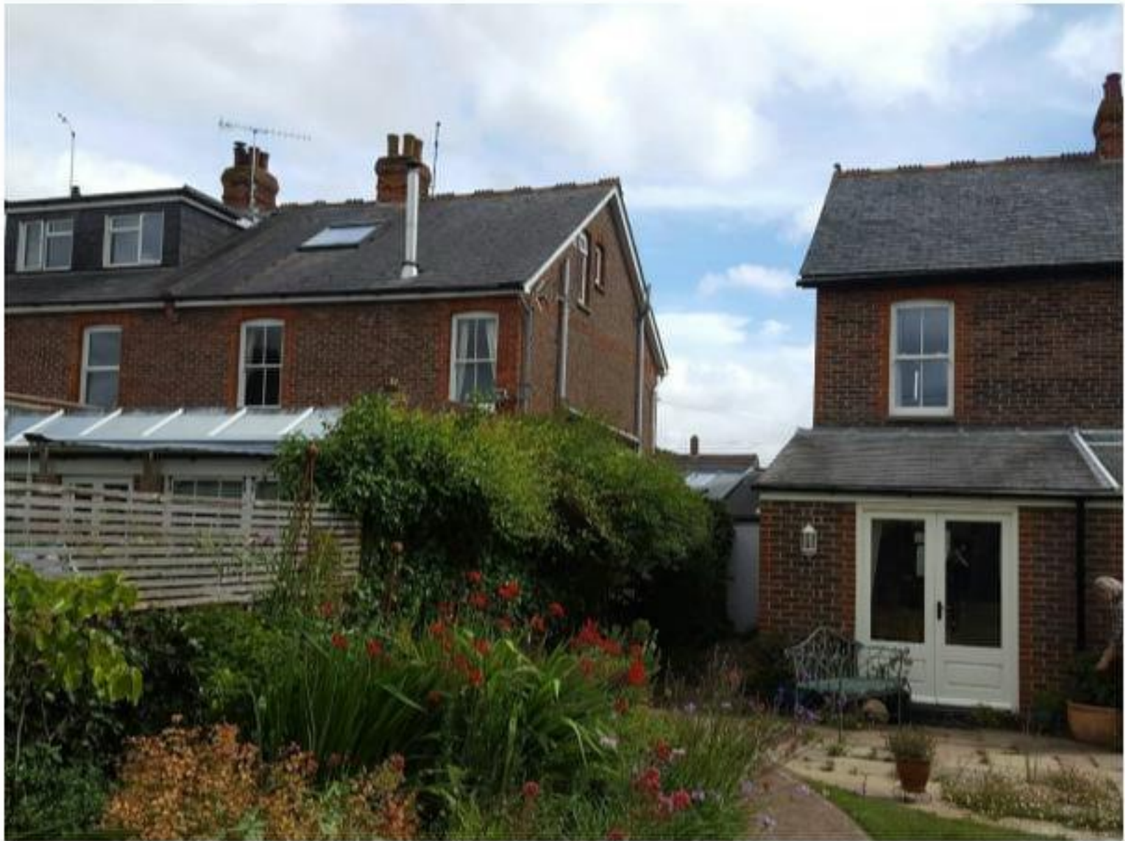
Photo 11: Rear of property where extension would be
