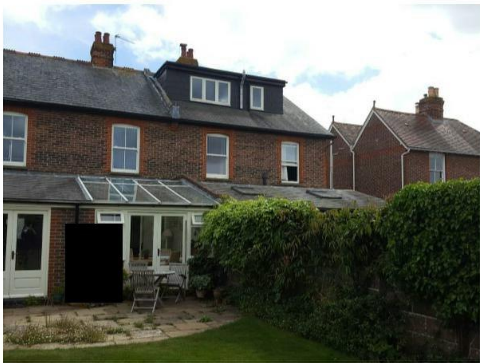
Photo 9: Rear of property
