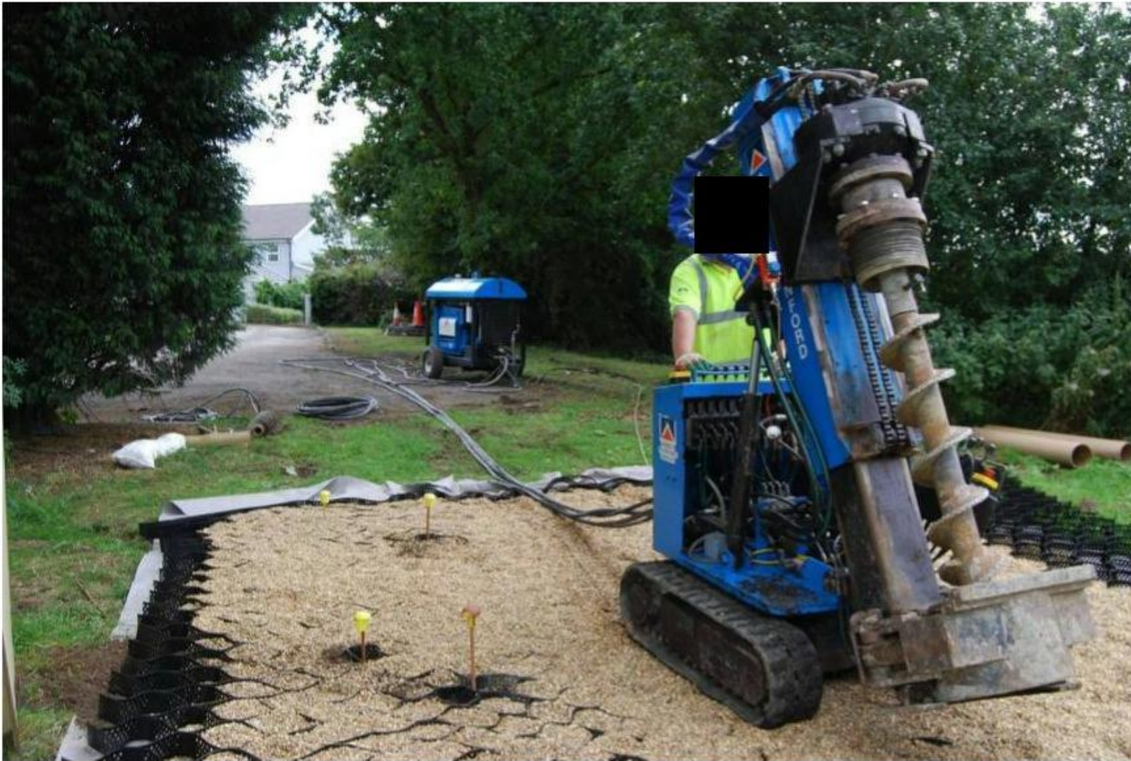
A typical piling rig used on a Tree Root Protection Service project. The rig is custom designed to have a very low bearing pressure, equivalent to a 12 stone man wearing size 10 shoes. The power pack (in back of photo) is left outside the root zone, leaving just the lightweight piling rig operating on the site.
