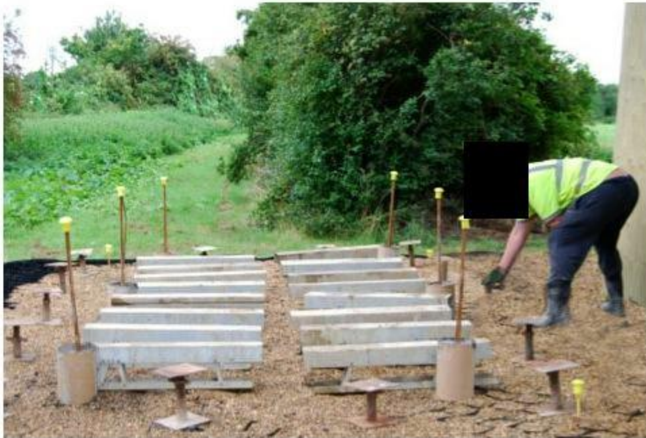
Perimeter jacks are laid around the edge of the footprint to allow fine level adjustments to be made.
