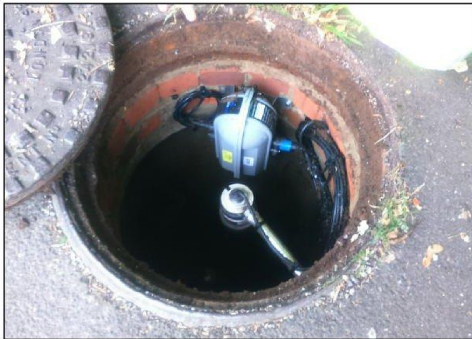
Figure 8: Photo of Southern Water Manhole 0801
