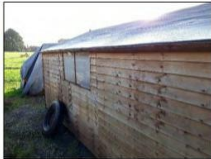
Figure 6: Bitumen felt roof and window of shed
