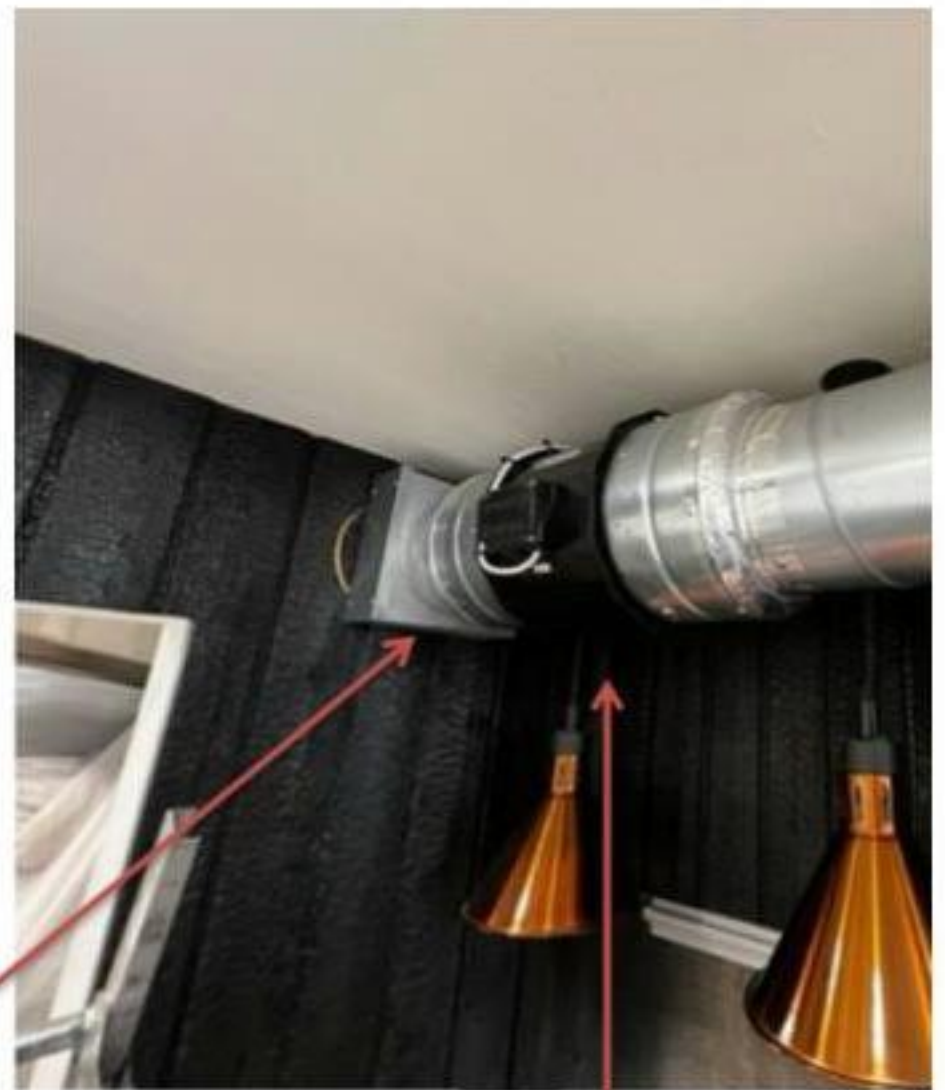
Boxed and sound proofed fan with access hatch for changing carbon filter
