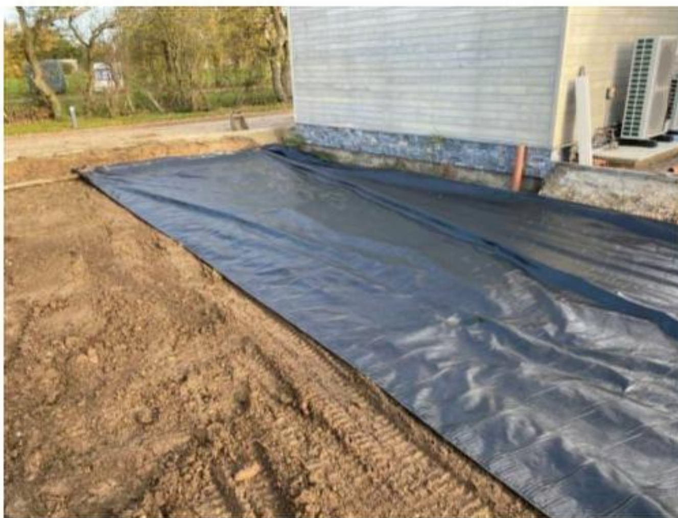
Photo 9: Excavation and geotextile prepared for topsoil placement (Photograph provided by Yachthaven)
