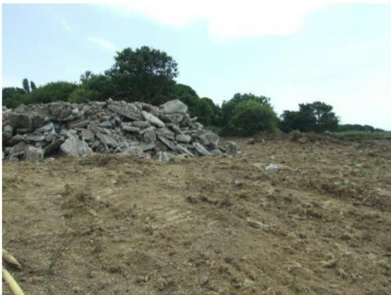
Photo 1: Demolition & site clearance as photographed in July 2018. Waste stockpiled ready for removal.
