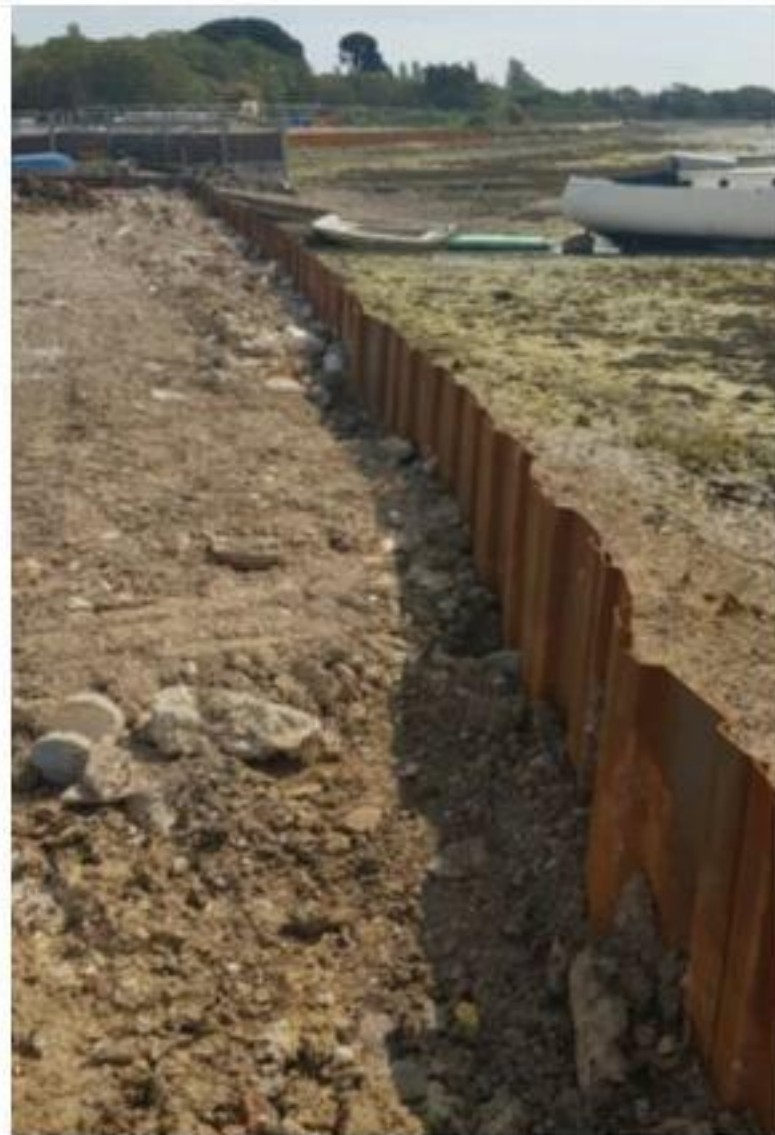
Photo 6: View of the completed sheet pile contamination migration barrier prior to capping & placing revetments (Photograph provided by Yachthaven).
