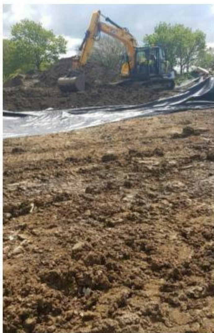
Photo 8: Excavation, geotextile placement and topsoil placement (Photograph provided by Yachthaven).
