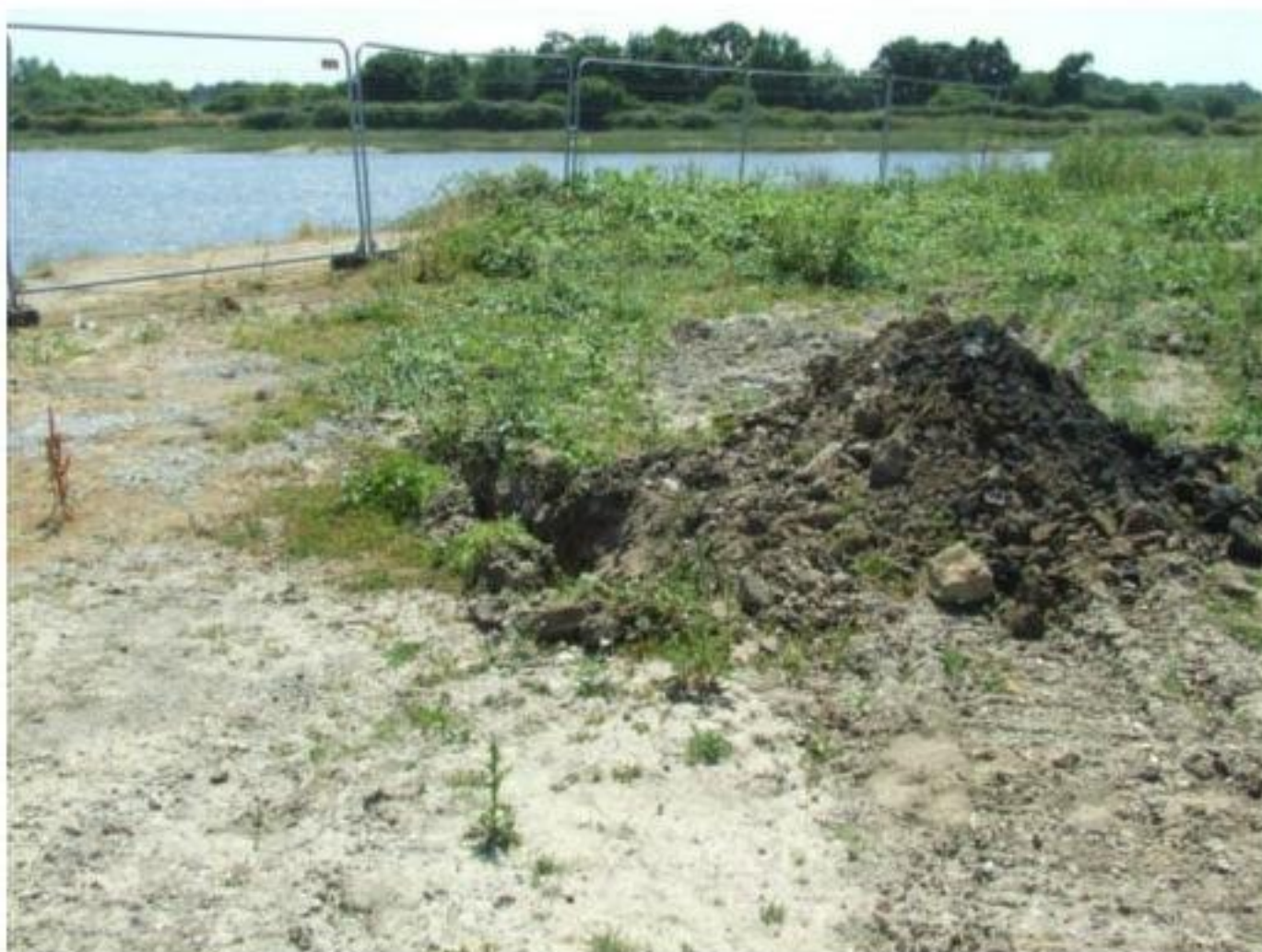
Photo 2: Typical trial pit excavated as part of the July 2018 site investigation.
