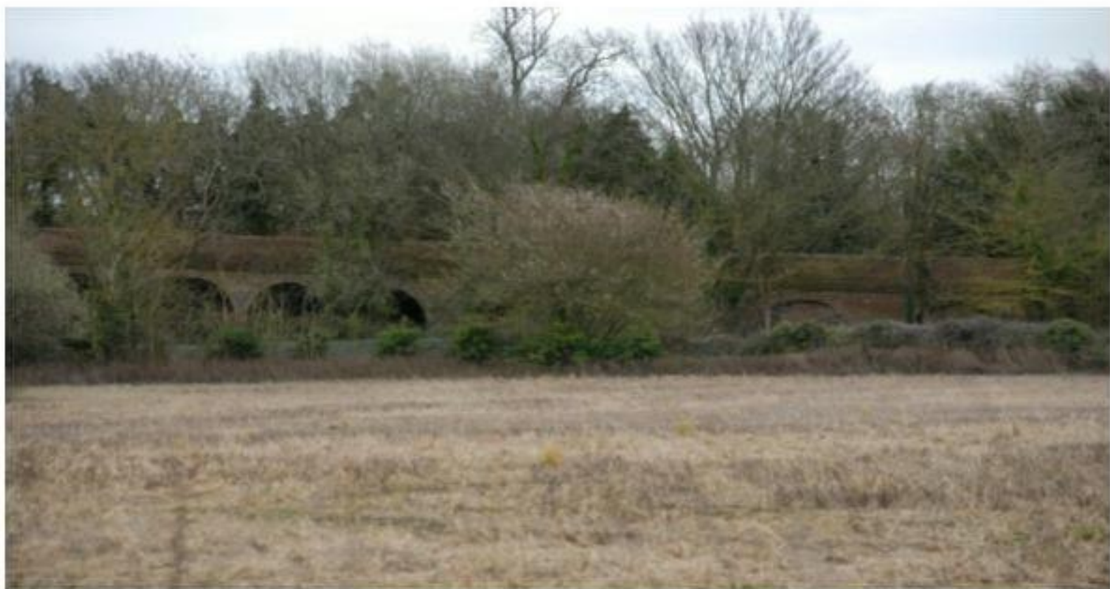
Mill Lane Bridge from Lower Road.
