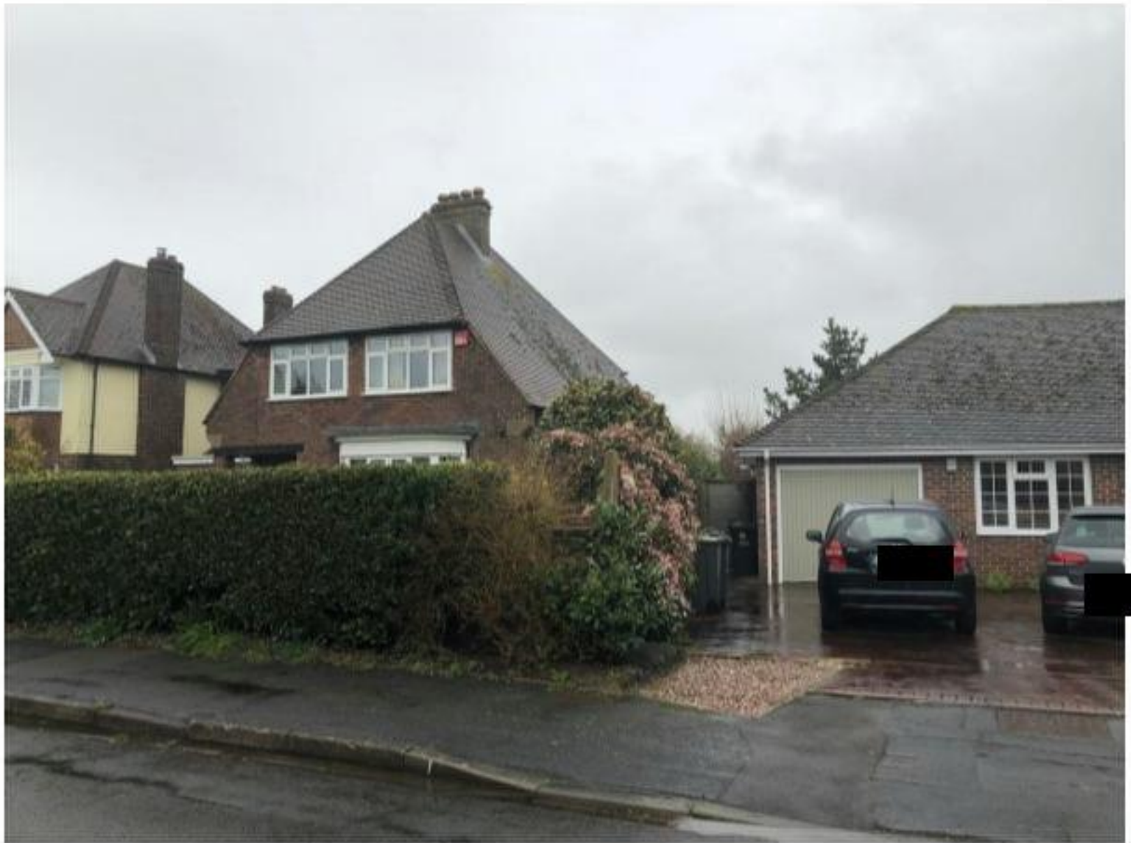
Photo 6: Front of the property showing No. 25 Clovelly Road
