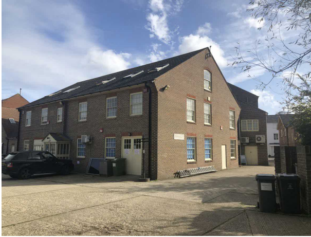
Figure 3: Rear of unit 3a.
