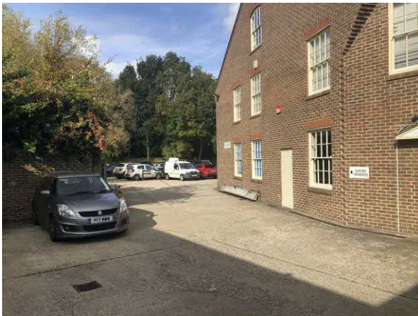
Figure 5: Existing access adjacent to unit (looking north).
