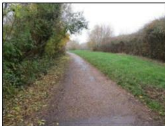
Figure 21: Tarmac footpath / cycle path Typical of Sections D and E
