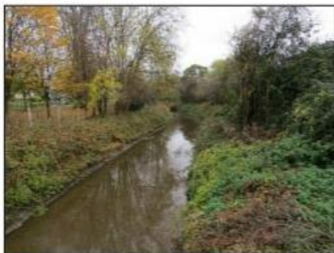
Figure 14: Hermitage Stream south of Corhampton Crescent showing concrete stream bed and banks
