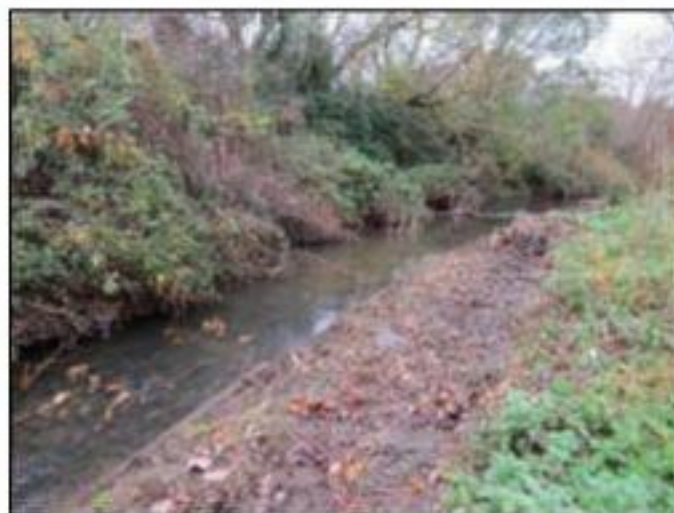
Figure 13: Hermitage Stream within Section D with concrete bed and oak weirs / edging
