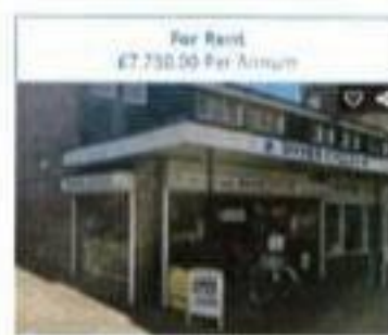
For Rent £7,750.00 Per Annum 10 North Street Arcade, Havant, PO9 1PX
