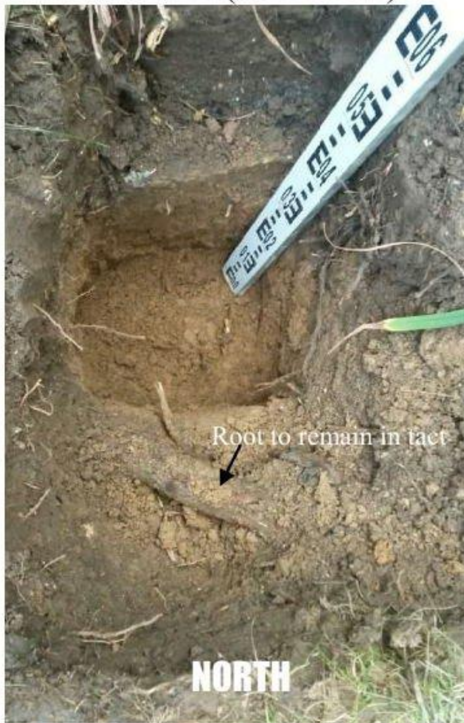
Trial Pit 1 (South West)
