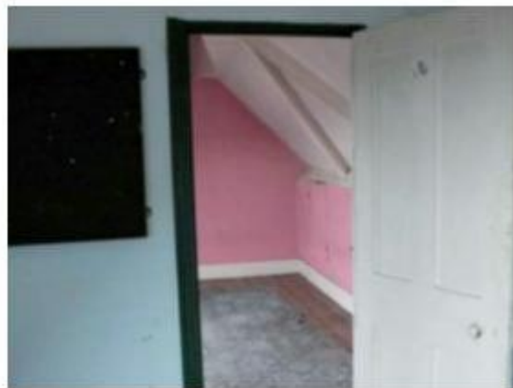
Second floor looking into west boundary room
