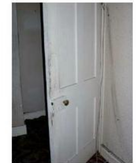
Four panelled doors throughout that have been boarded one side
