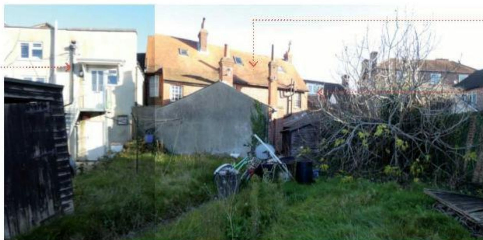
View looking towards rear elevation of property
