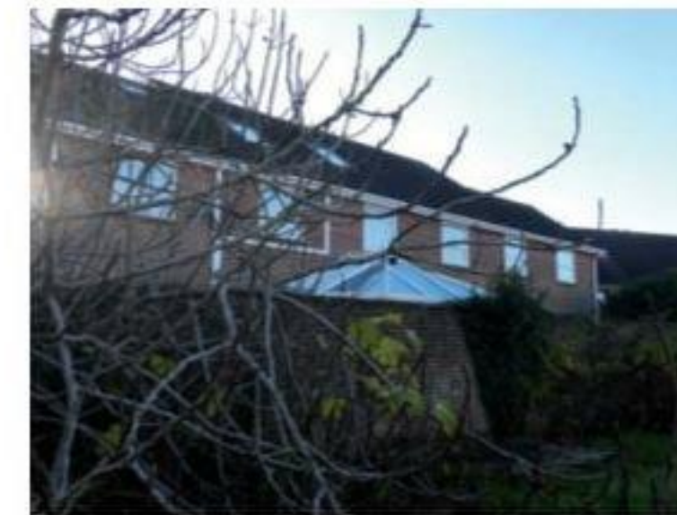
Rear elevations of 1D and 1E School Lane; conservatory on the ground floor and rooflights
