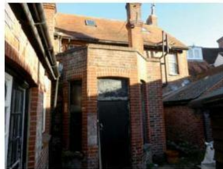
Looking towards rear elevation of property
