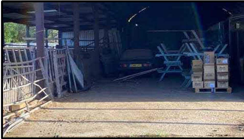
Golf centre driving range balls on their pallet and the Tee Caddy Café outside benches in the background. Storage of an old ford capri. There does not appear to be any planning permission consent from HBC for using barn 2 for any other use than agriculture. Photograph date 20/08/2020
