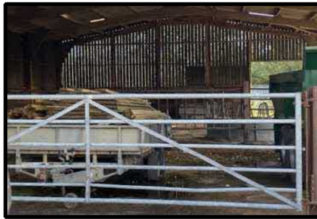
As above. Photograph date 28/07/2021
