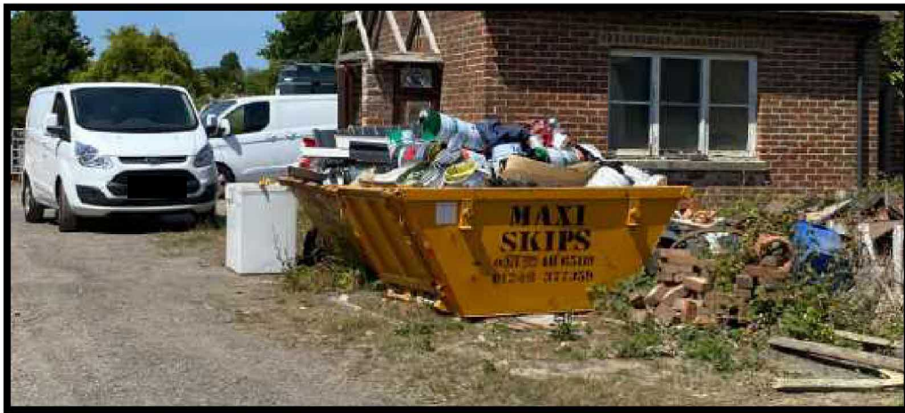
Smartline Southern vans loaded up with new materials and disposing of waste in their skips. Photograph date 02/06/2020
