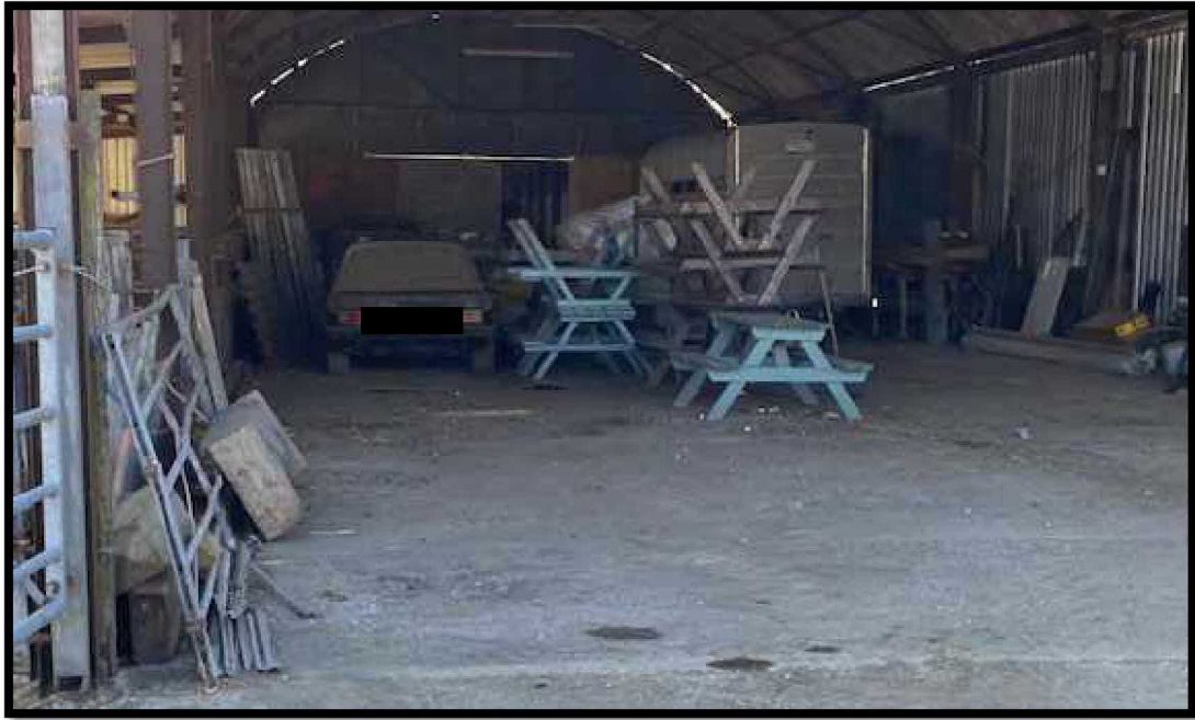
The Tee Caddy Café outside benches being stored. Storage of an old ford capri. There does not appear to be any planning permission consent from HBC for using barn 2 for any other use than agriculture. Photograph date 16/04/2021
