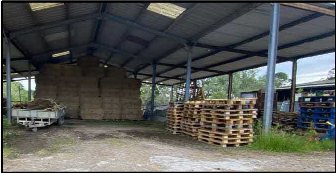
Haybales being stored at rear of the barn. To the left is a large trailer loaded with decking planks – not agricultural use and believed to be for Phillips Fencing and Landscapes business. To the right are the store of used pallets from Phillips Fencing and Landscaping and Smartline Southern. Photograph date 15/07/2021
