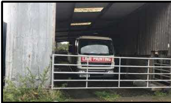
Smartline Southern line marking lorry being stored in the South barn 3 Lean-to. This is not agricultural production or use. No planning permission request or grant for this change of use appears to exist at HBC. Photograph date 04/10/2019
