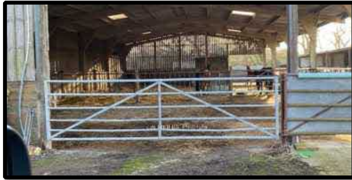
No cattle present, the southern end of the barn is being used by three horses (not agricultural use). Photograph date 09/01/2022
