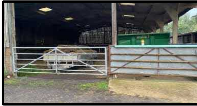
Phillips Fencing and Landscapes trailer loaded with wooden decking. Not agricultural use. There is no HBC consent for change of use of this barn from agricultural use. There are no cattle present. Photograph date 25/07/2021
