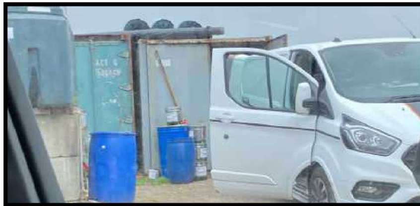
Another day and another unloading of waste and refilling vans with new materials. Photograph date 31/03/2021
