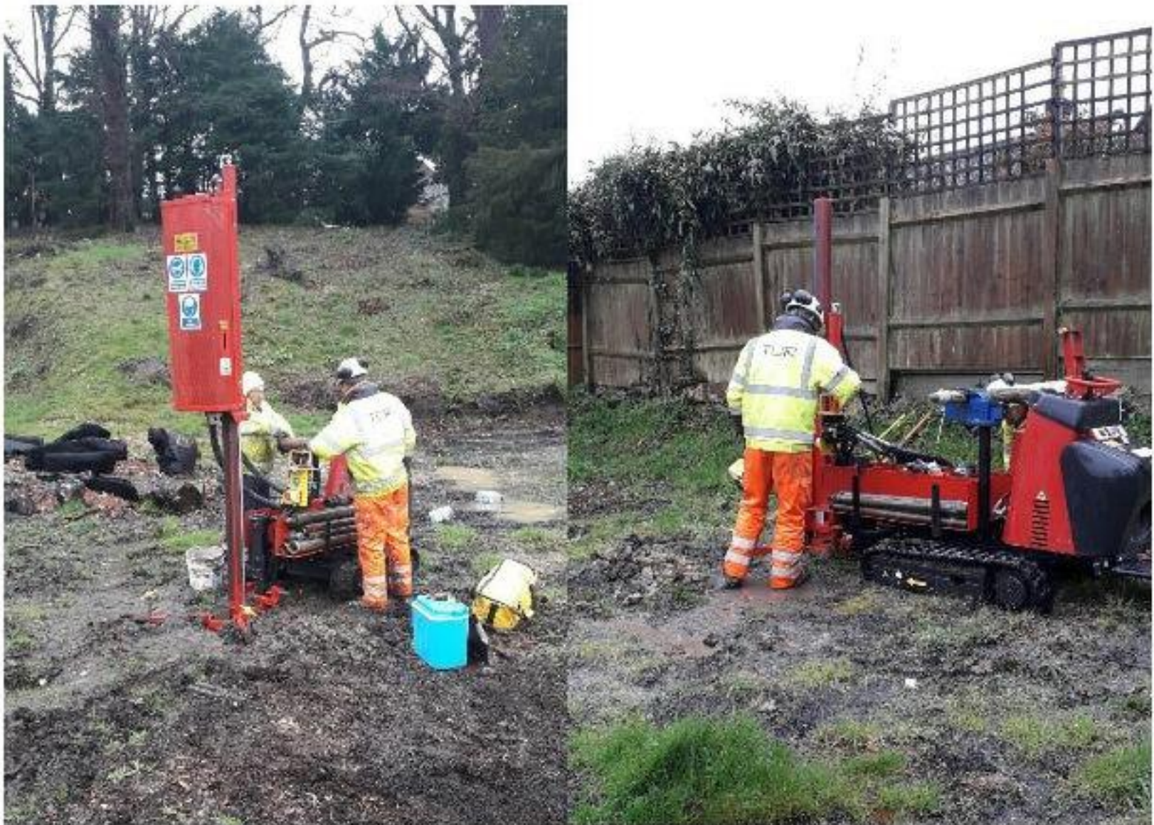
Plate 2: Drilling WS201 (left) and WS202 (right).
