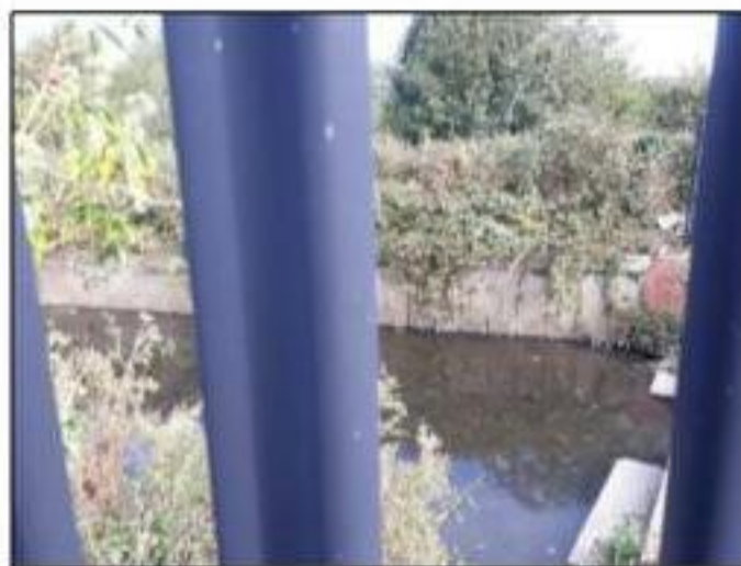
Figure 7: Artificial banks along Hermitage Stream abutting the western site edge
