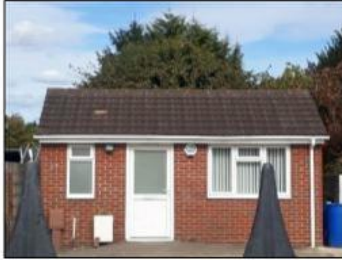
Figure 5: Office building at 178A West Street
