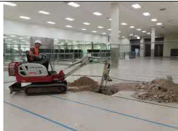
Photo 9: Trial pit excavation within building towards the northeast of the site.
