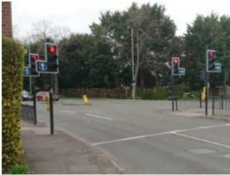
Photograph 13: Signalised junction of Bedhampton Road/Hulbert Road
