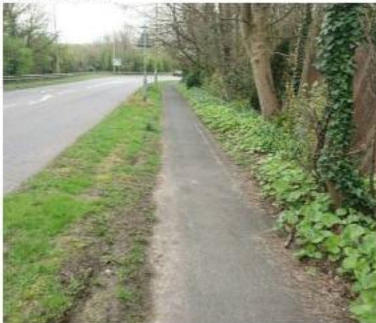
Photograph 21: Pedestrian footway along northern side of Bedhampton Hill
