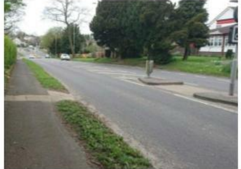
Photograph 14: Pedestrian Refuge Island crossing on Bedhampton Road
