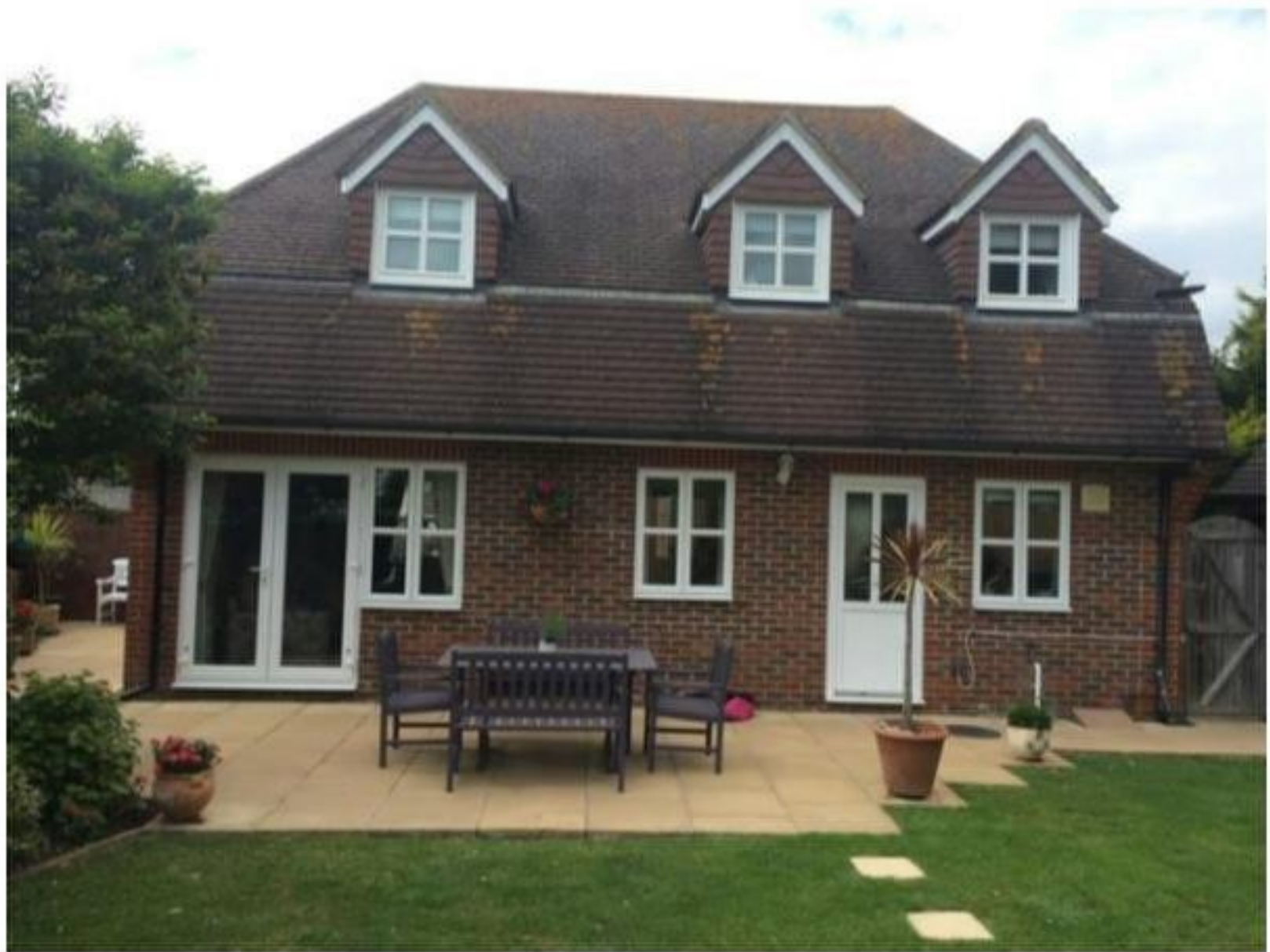
Photo 7: Rear Garden looking west and rear elevation of house
