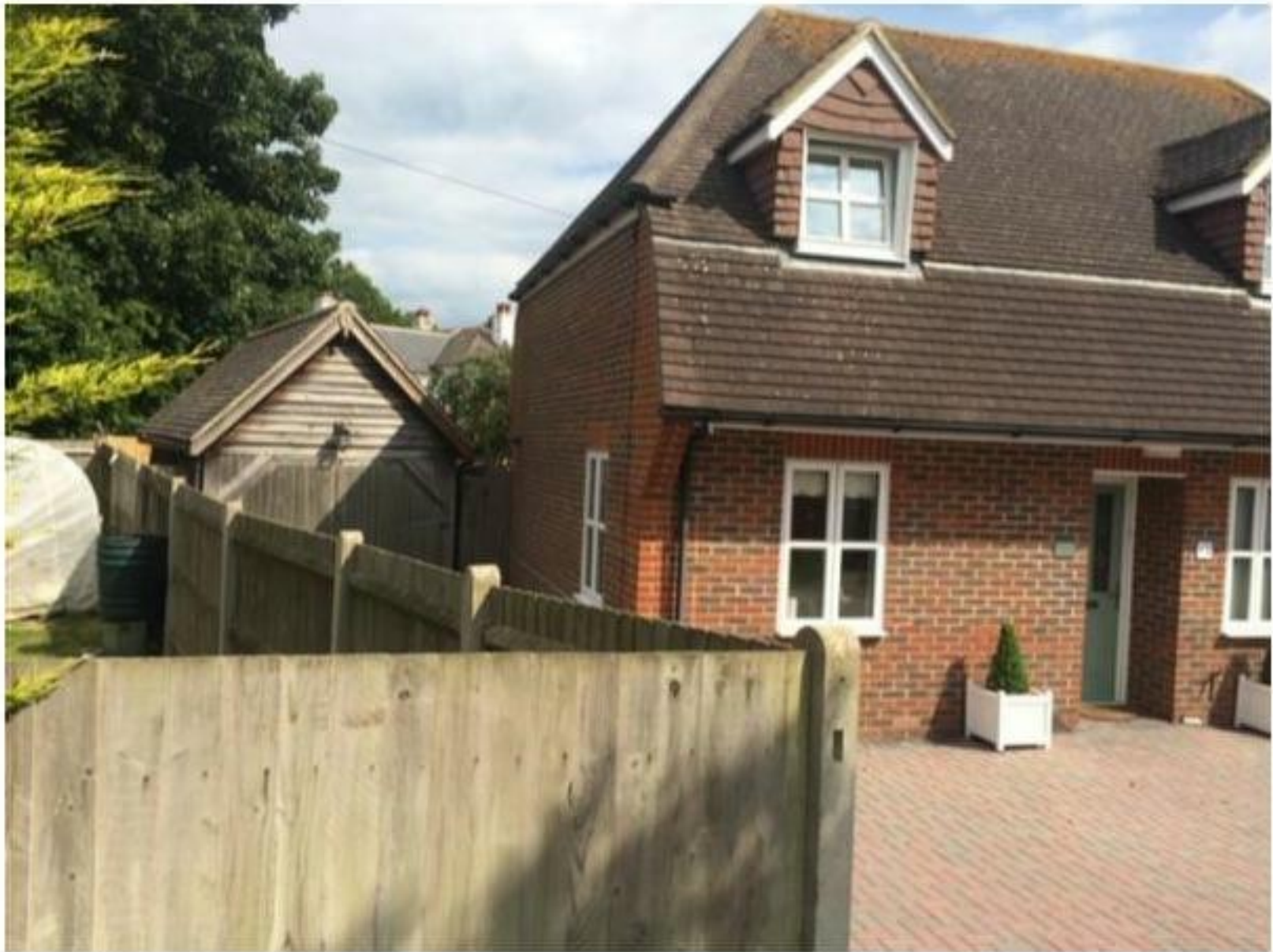
Photo 4: Northern side elevation showing garage
