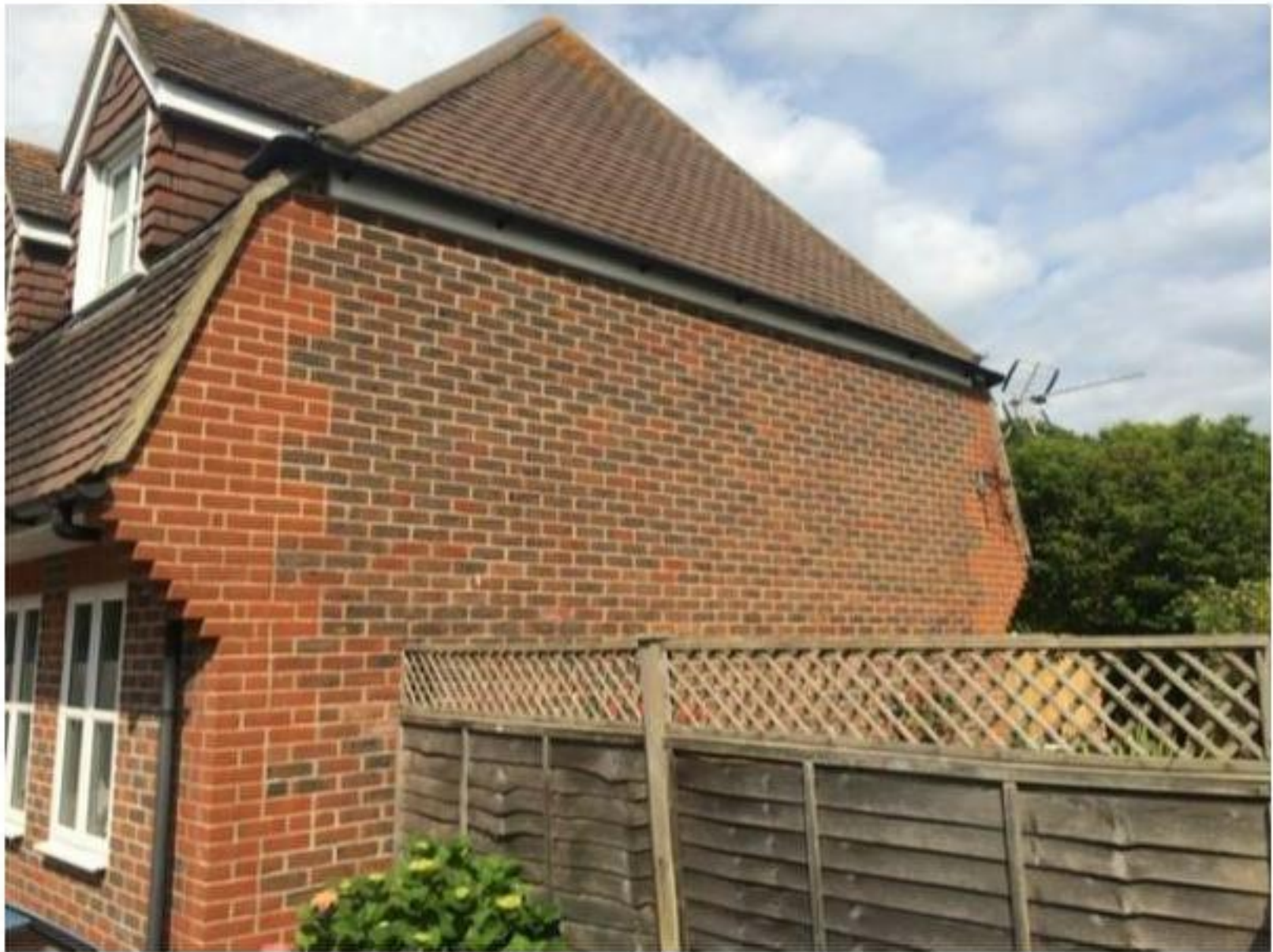
Photo 8: Southern Side Elevation
