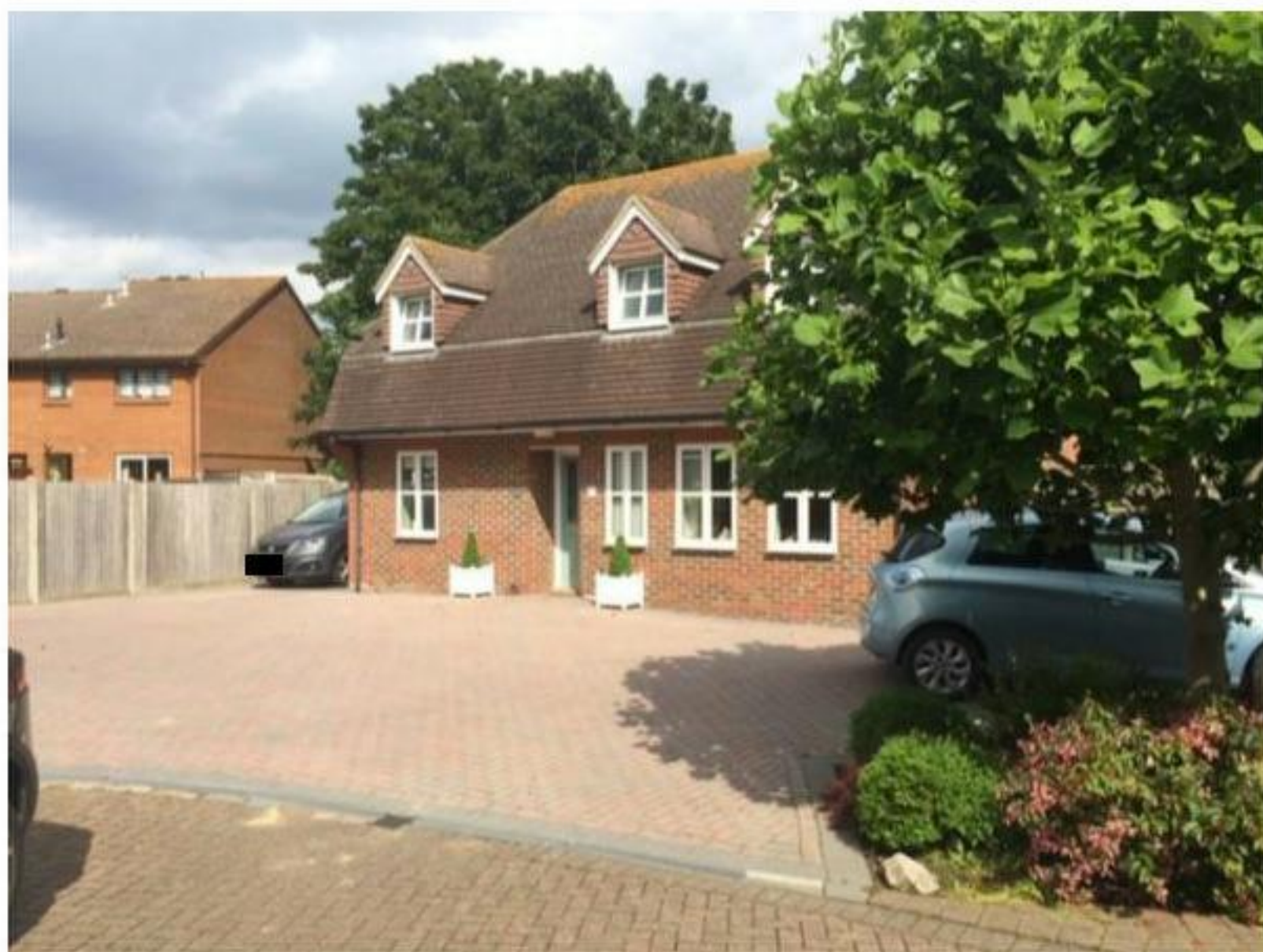
Photo 9: West elevation showing forecourt
