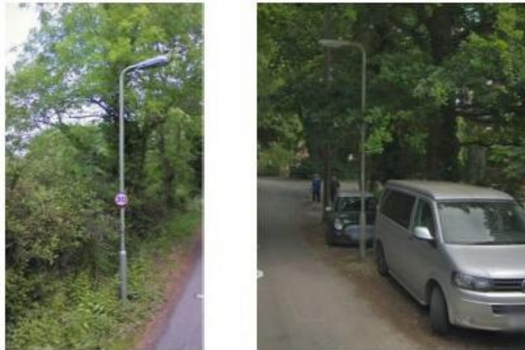
Figure 5-2 – Typical lighting installed along Long Copse Lane
