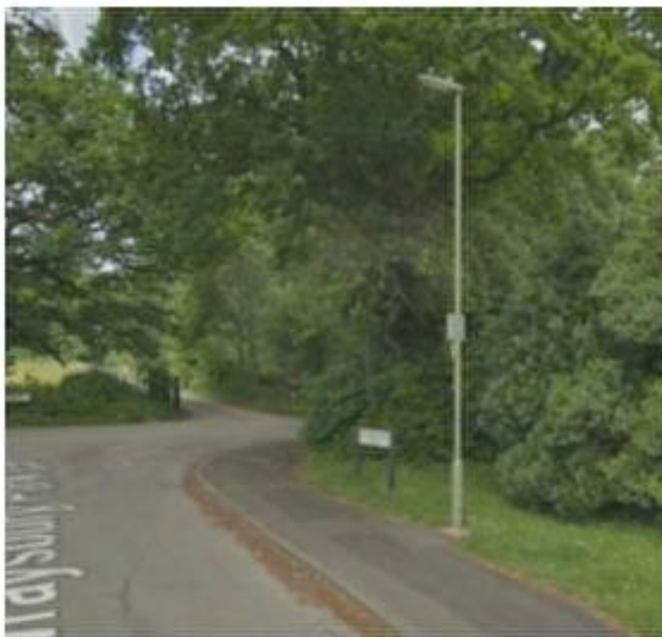
Figure 5-1 – Typical post top mounted type lighting in residential areas
