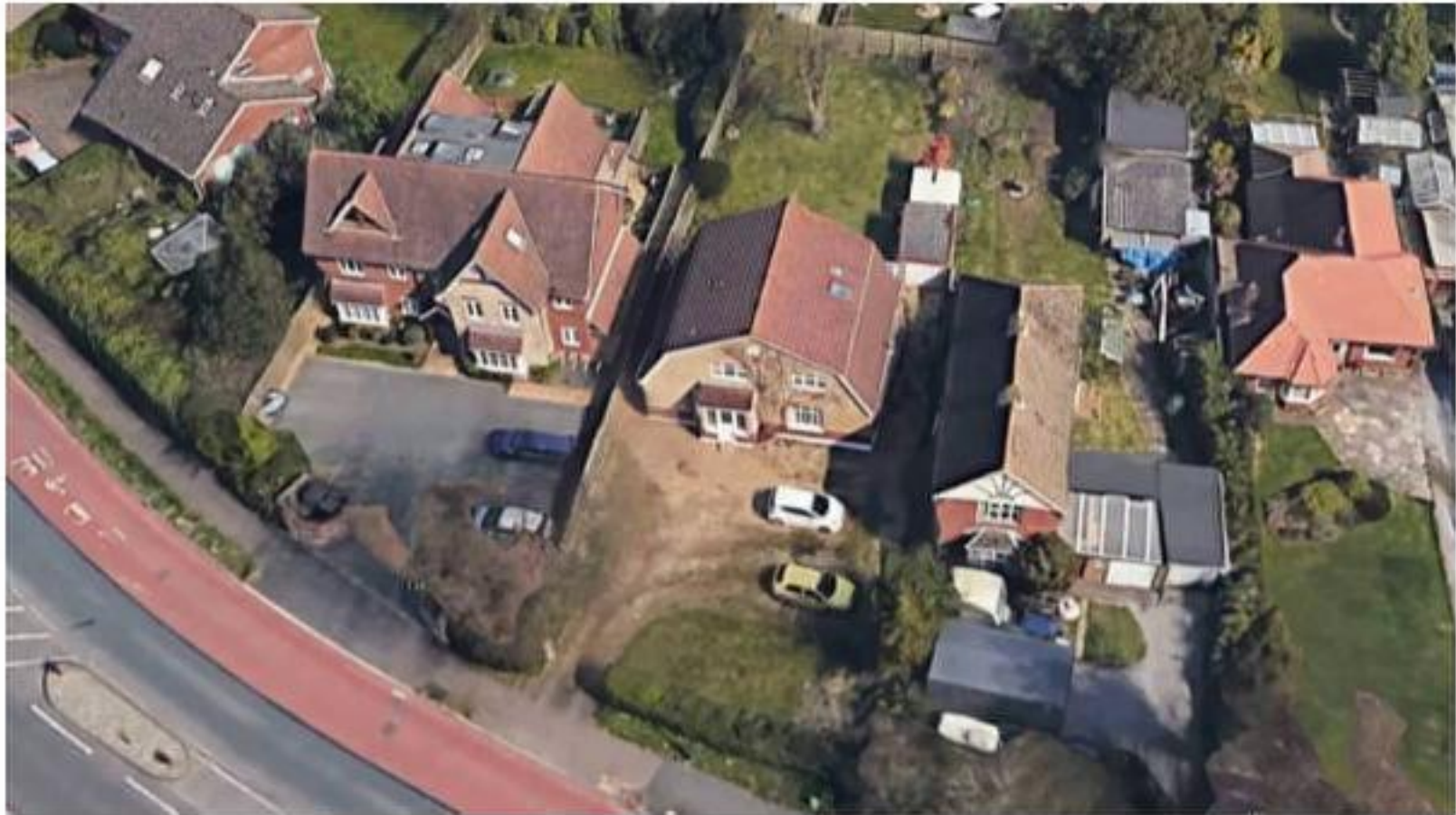
Above, aerial image looking east and showing the front elevation and boundary of the property.
