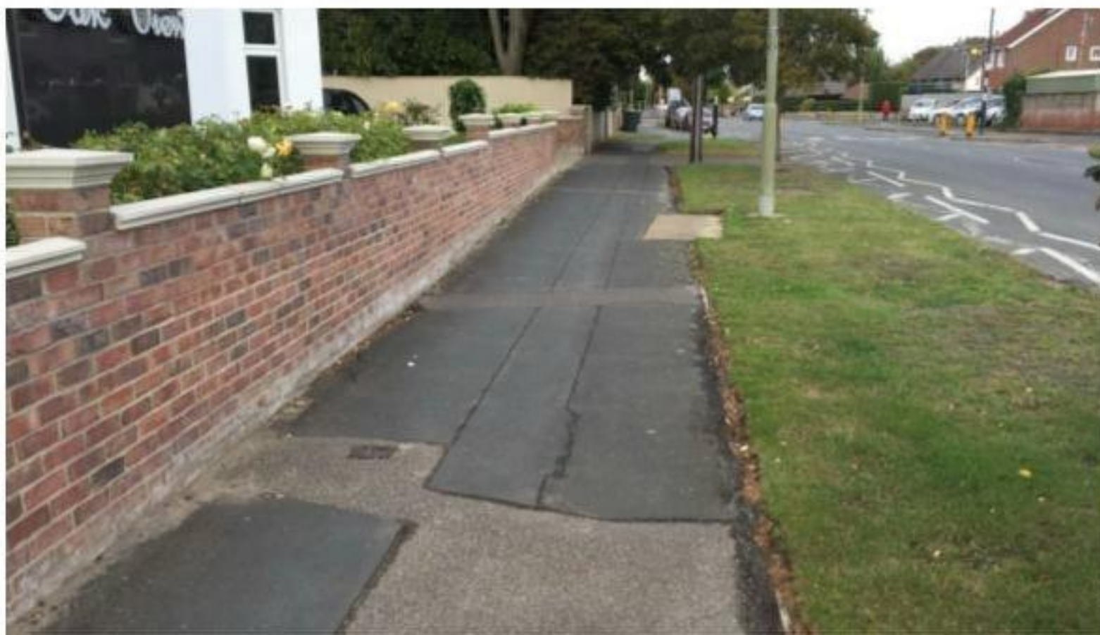
Footway Flanking Beach Road
